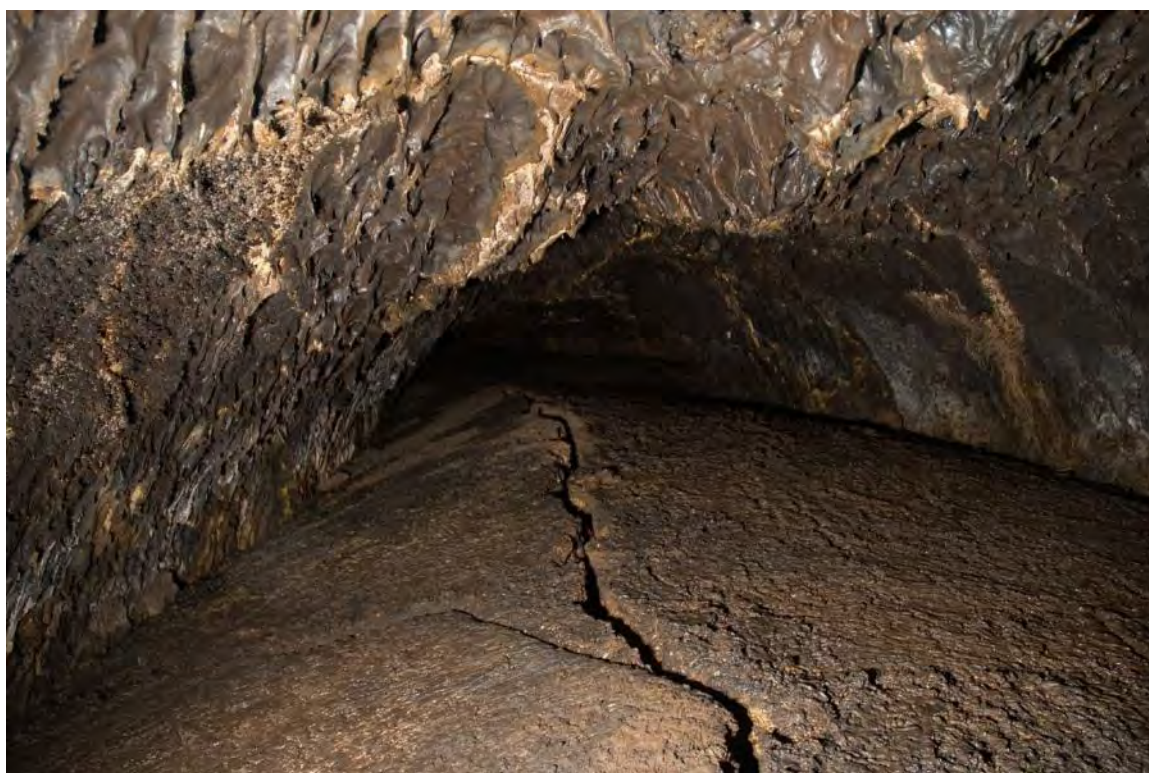
Figure 7. Contraction cracks in Catacombs Cave.
