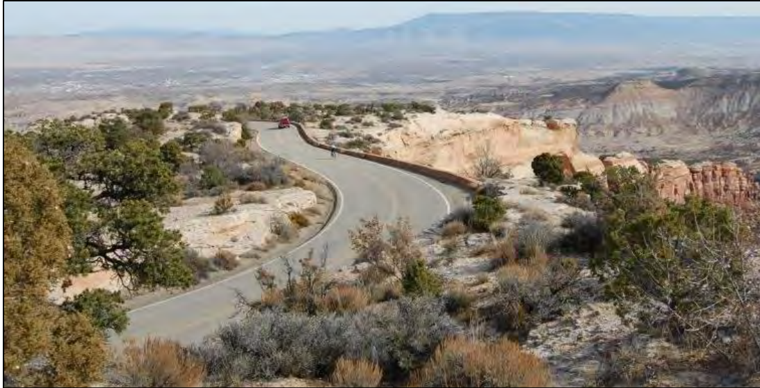
Photo 1. Rim Rock Drive (NPS photo).
