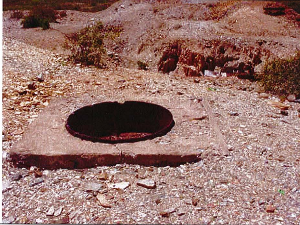
7. Chimney foundation located on the east side of the main mining pit.
