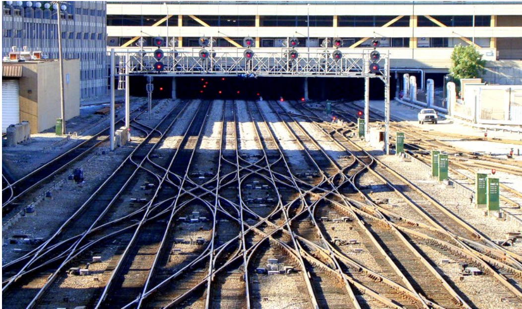
Figure 16. Control points approaching Chicago Union Station
