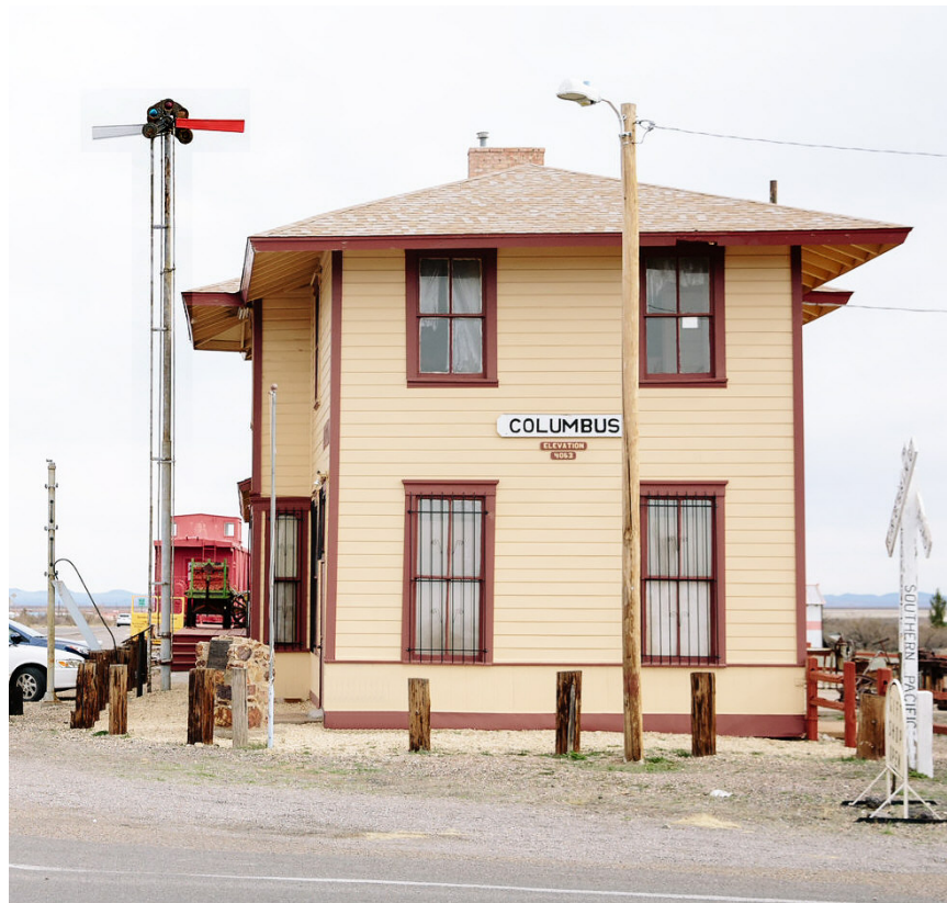
Figure 18. Columbus, N.M. restored railway depot
