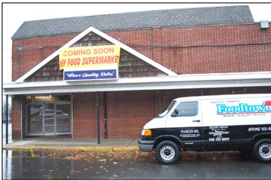
The sign for Key Food Supermarket adorns the former South Amboy Foodtown building, and seeing that the new store will be open soon, has made many local residents very happy to do know they will be able to do their grocery shopping in town once again. According to inside sources, the store is expected to open sometime in March. (Photo by Tom Burkard)
