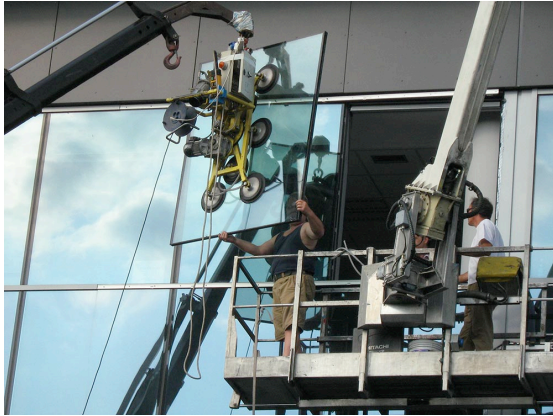
Figure 2 - Installation of a modular panel
