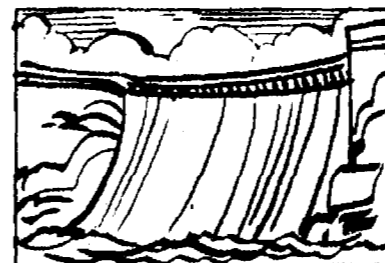
During the construction of the Hoover Dam, concrete had to be poured continually for two years.
