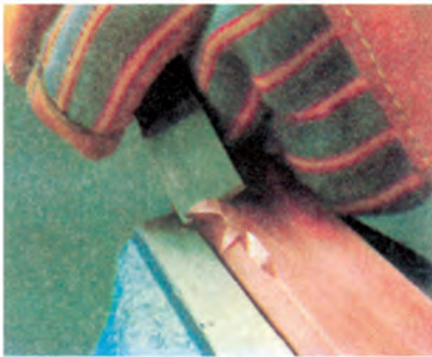
21 Scraping metal surfaces
