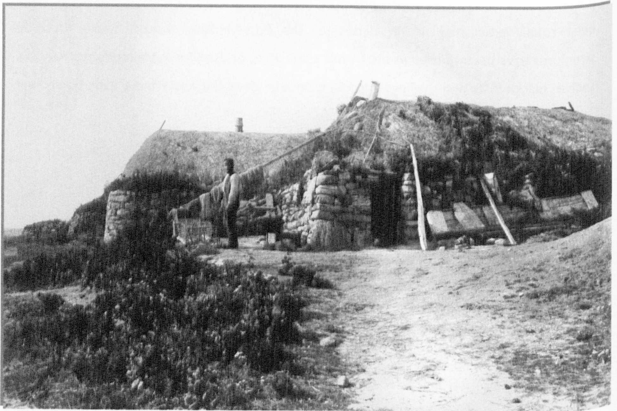
Figure 5.4 Hogarry, North Uist - photo by Erskine Beveridge taken in 1904. The opportunistic reuse of ancient drystone structures in the Western Isles was endemic. This is understandable in light of the limited sources of alternate materials.
