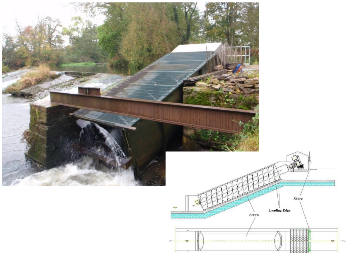
Figure 2.2 Hydraulic screw turbine in place at Howsham Mill and schematic of Archimedes screw turbine shown from the side and above (inset; MannPower Consulting).
