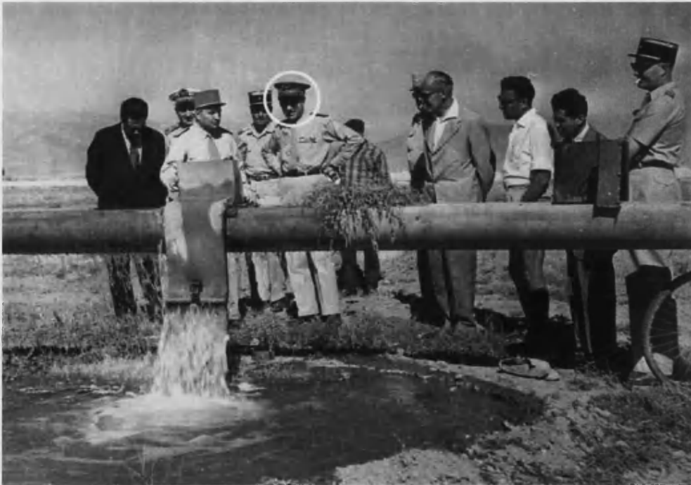
17. Inspects new irrigation works...
