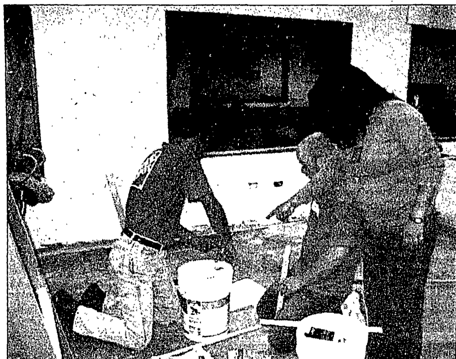
The expansion of the Niles Teen Center was mostly completed June 11 after several days of work from more than a dozen volunteers from Home Depot. (Photo courtesy of Niles Teen Center)
