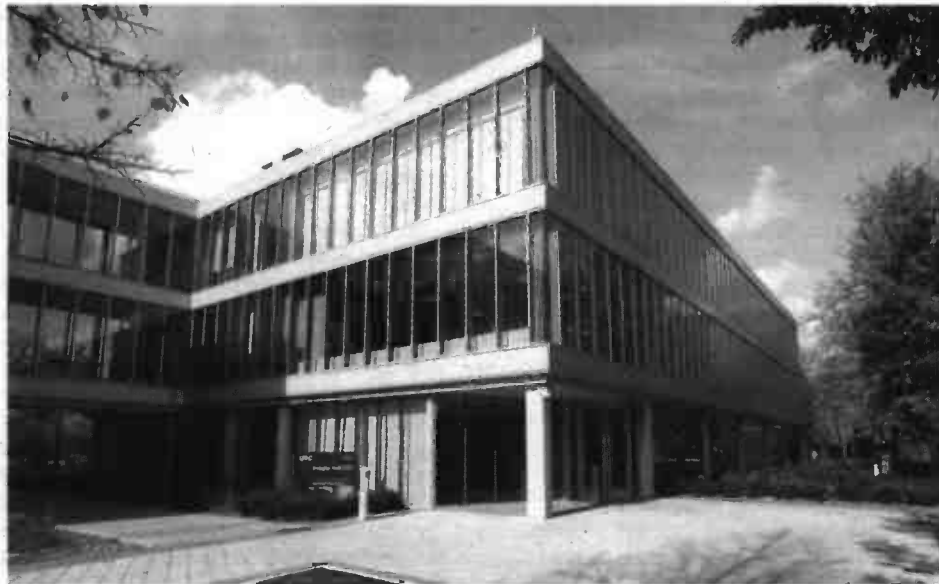
Old and new: Although The University of Illinois at Chicago's Douglas Hall was built in the '60s, its recent rehab added solar energy panels, automated interior lights and water savers. The building houses the College of Business Administration. I SUPPLIED PHOTO
