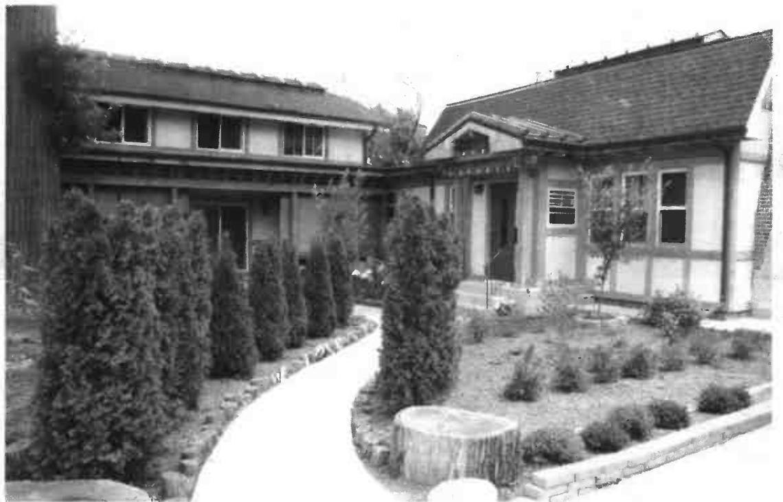
Morton Grove officials decided that Soon Yoon has to reconstruct her newly renovated house to fit into a footprint that's 10 feet smaller. | RICK KAMBIC/SUN-TIMES MEDIA
