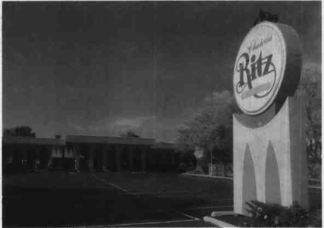
The exterior of Chateau Ritz isn't flashy, but that belies the often-renovated interior of the Niles banquet hall. | IGOR STUDENKOV/FOR SUN-TIMES MEDIA
