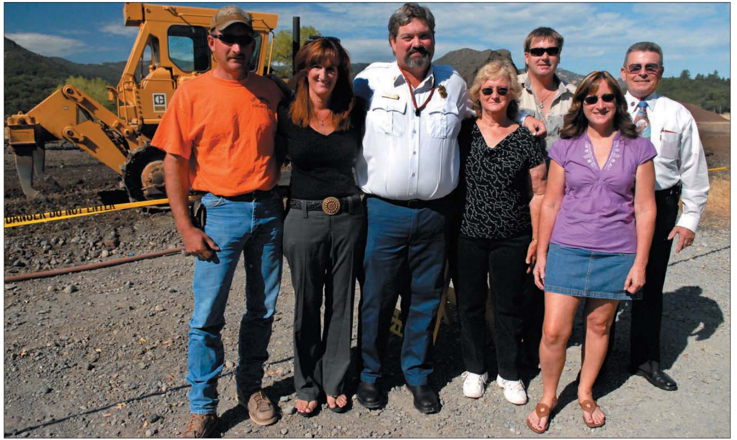
Mike Lucchetti, Rena Trimble, Hoss Milone, Rose Lucchetti, Bruce Jensen, Barbara Green and Wesley Clark gather for the start of construction at the site of the new Hopland fire station.
