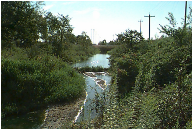
Process and Stormwater Flow Near Outfall K001 - 1999
