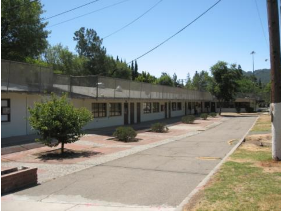
Photograph 9: Classroom building and attached Principal's Office (at far end). View looking south.
