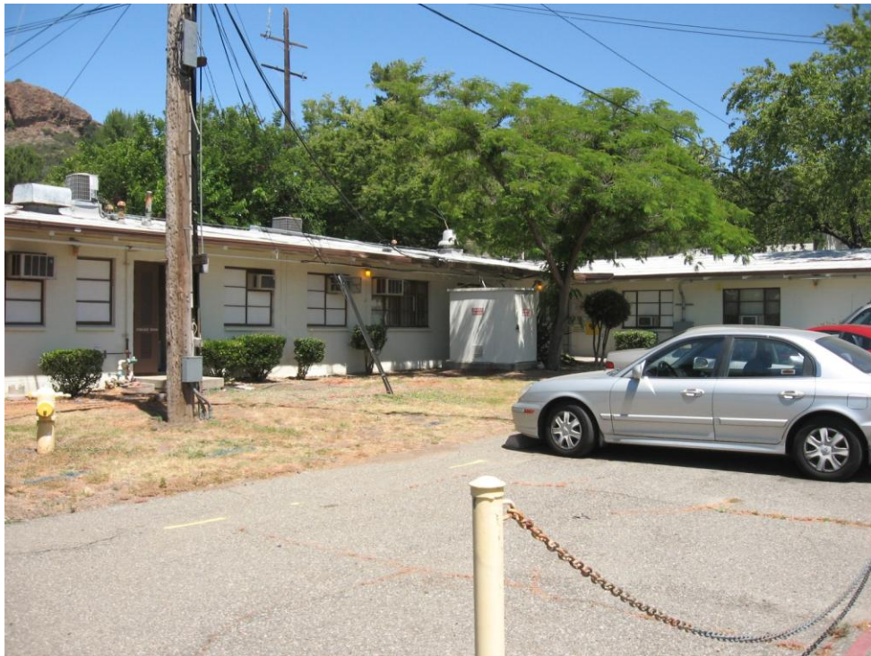
Photograph 12: Administration Building. The original Administration building is the left wing, the right wing was added in 1973. View from main driveway, looking northwest.
