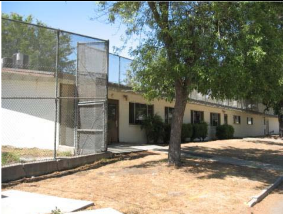
Shared Kitchen and Mess Hall. View looking west.
