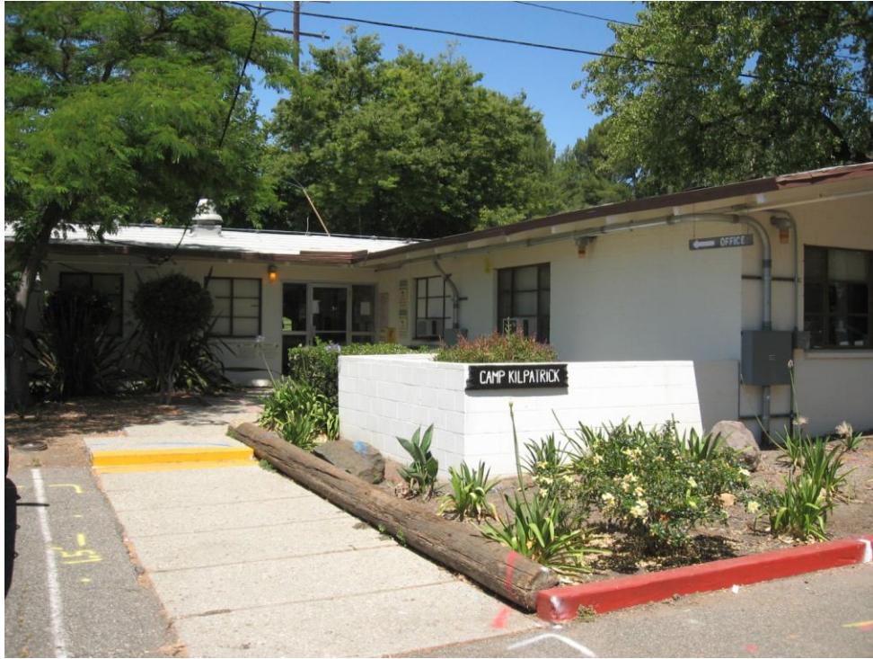
Photograph 13: Administration Building entrance. The Administration wing to the right was constructed in 1973. View from main driveway, looking west.
