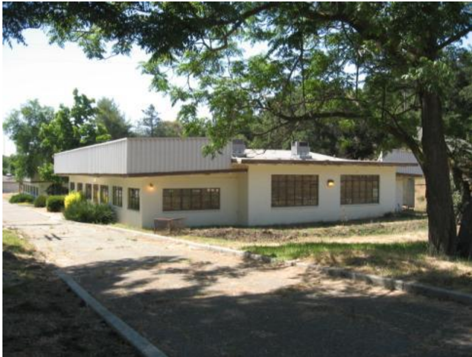
Photograph 4: 40-Bed Dormitory 1A. View looking southwest.
