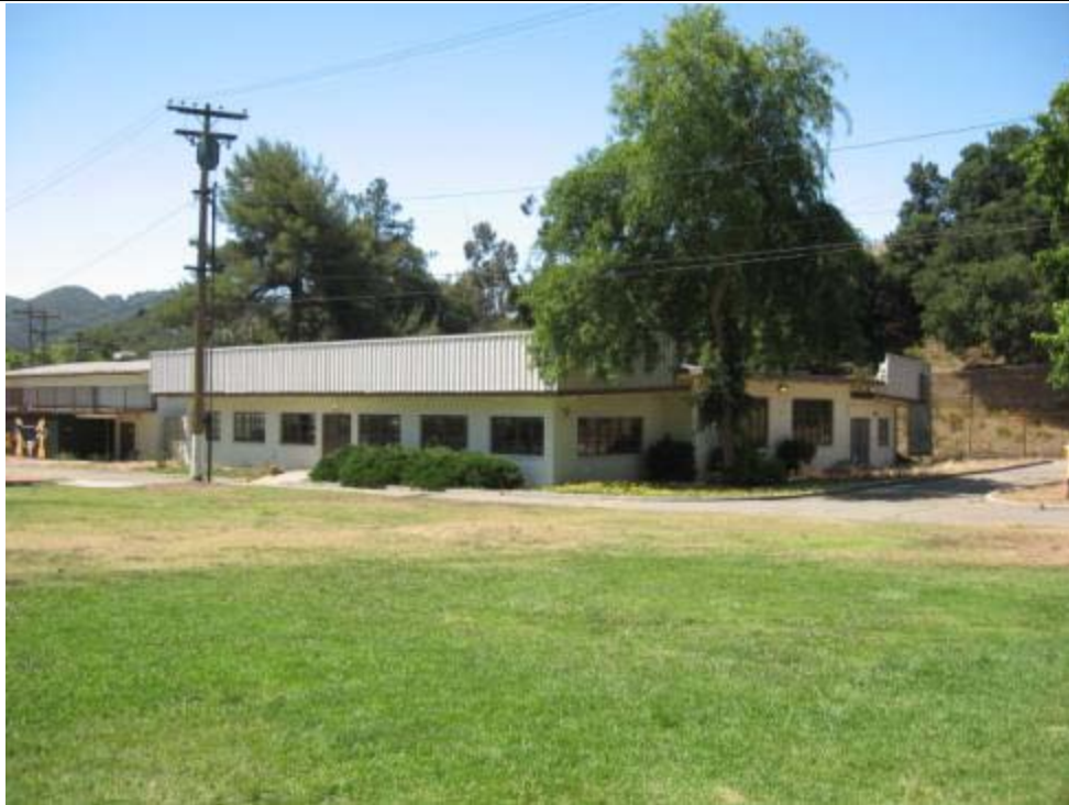
40-Bed Dormitory 1B. View looking southwest.
