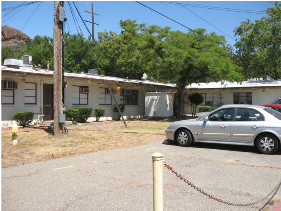
Administration Building. The original Administration building is the left wing, the right wing was added in 1973. View from main driveway, looking northwest.
