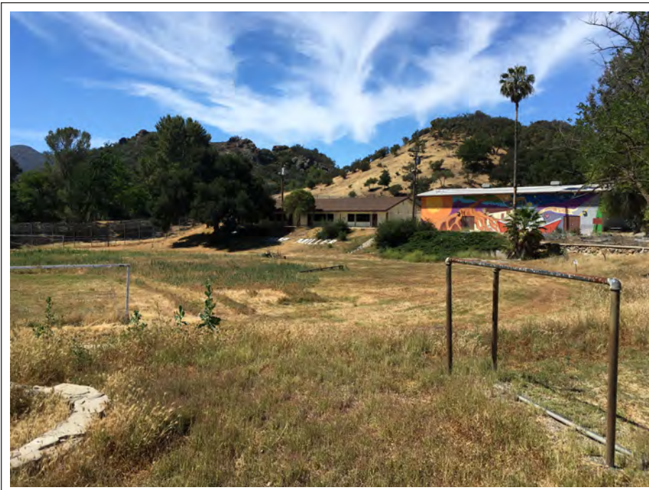
Photo Location 8. June 2018. View of conditions in Camp Miller where recycled water line will be installed.
