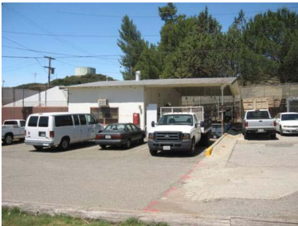
Maintenance Building and Garage. View from main driveway, looking west.
