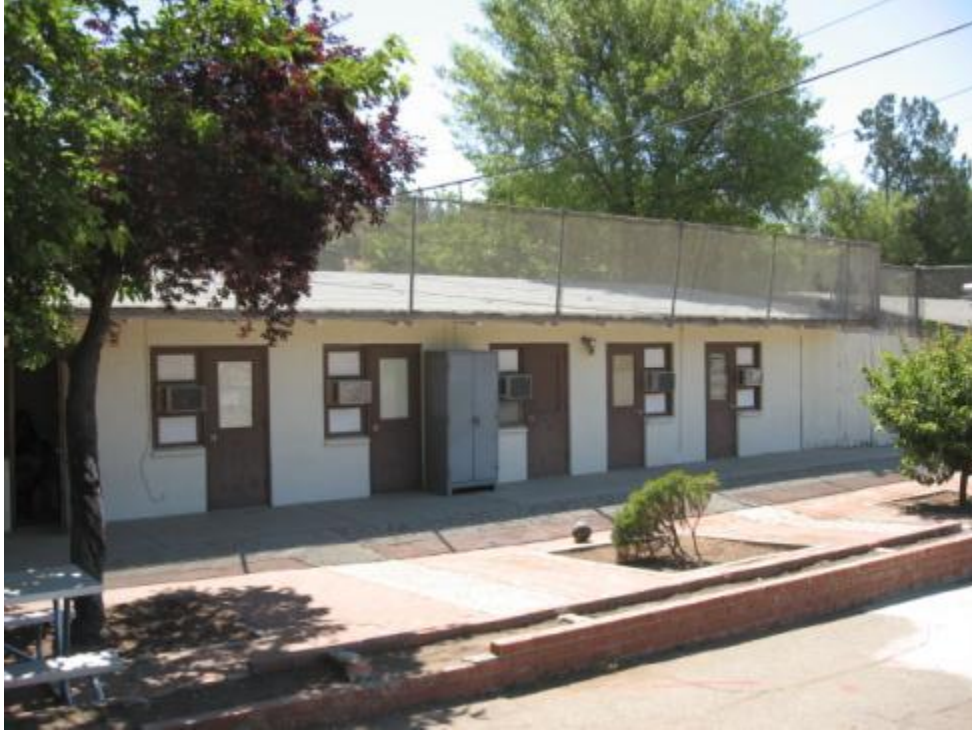
Photograph 11: Counselor offices in Administration Building, added in 1963. View looking southeast.
