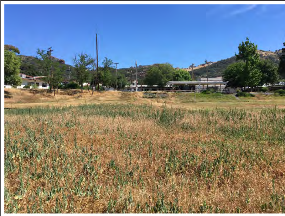
Photo Location 7. June 2018. View of conditions in Camp Miller where recycled water line will be installed.
