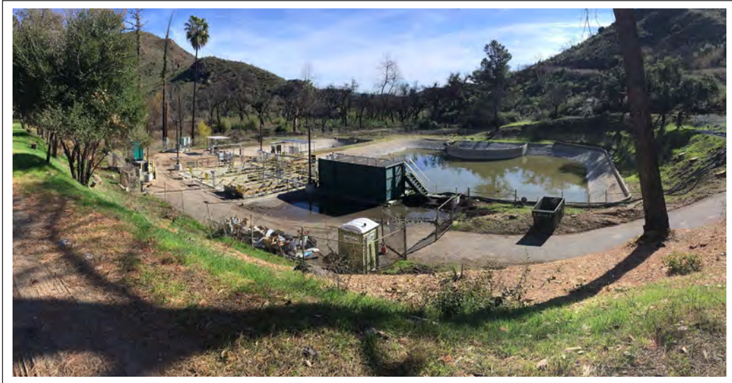
Photo Location 5. January 2020. Overview of permanent wastewater treatment plant project site.
