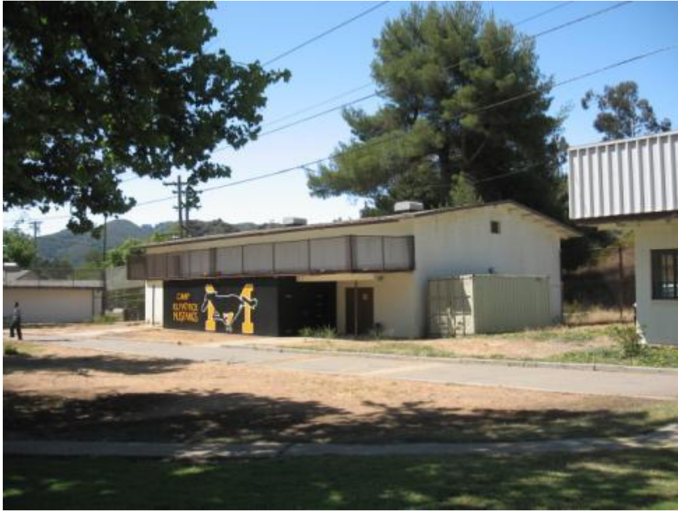
Photograph 7: Gymnasium. View looking southwest.
