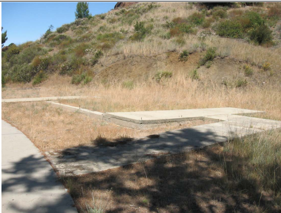
Foundation pad of demolished "comfort station" located to the east of the swimming pool. View looking northwest.
