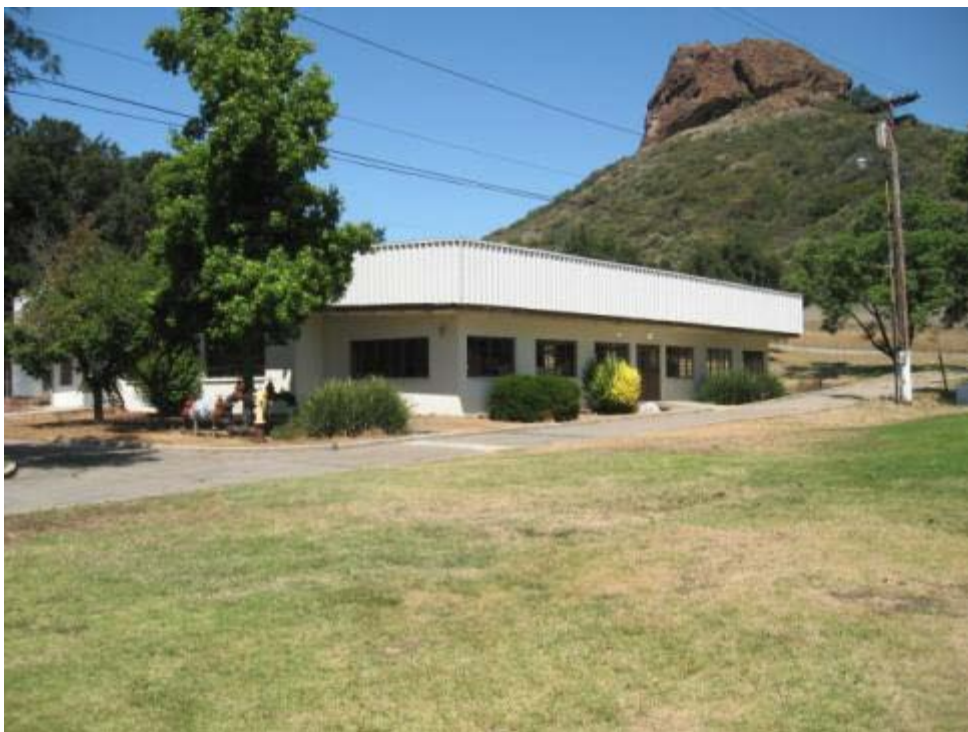
40-Bed Dormitory 1A. View looking northwest.
