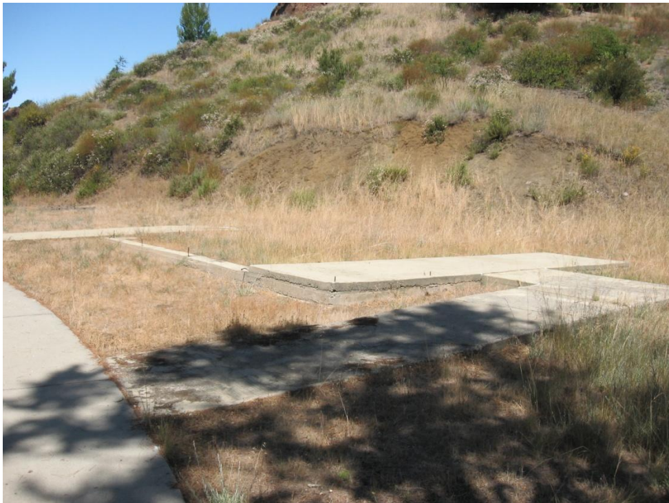
Photograph 18: Foundation pad of demolished "comfort station" located to the east of the swimming pool. View looking northwest.
