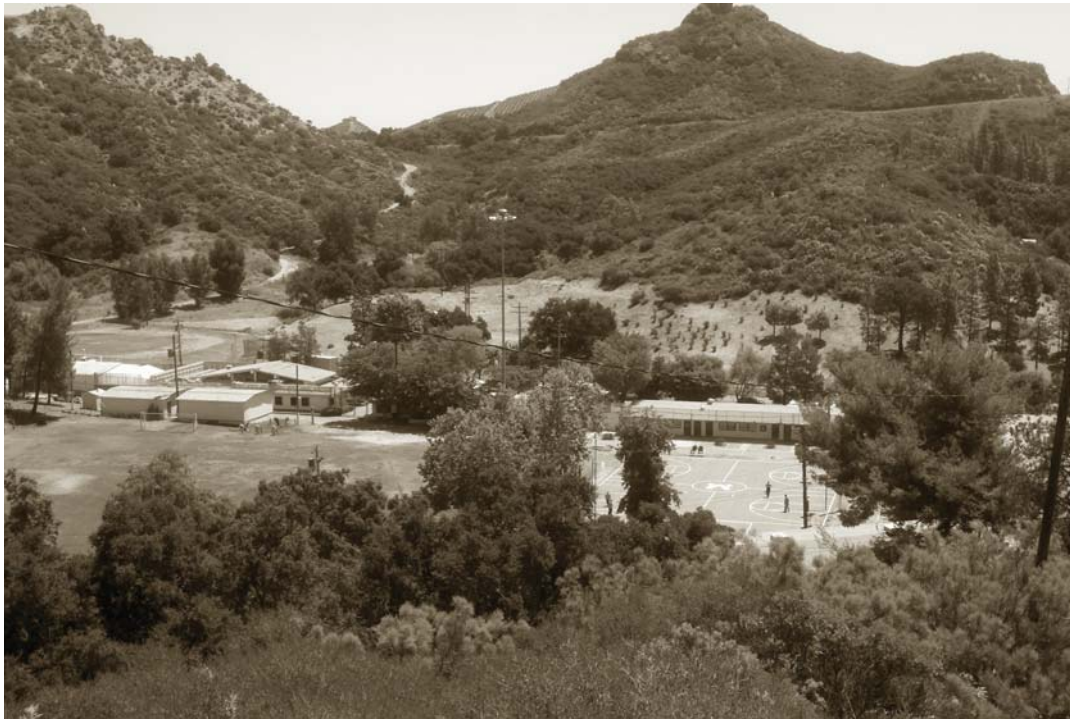
Camp overview from Water Tank: Looking east.
