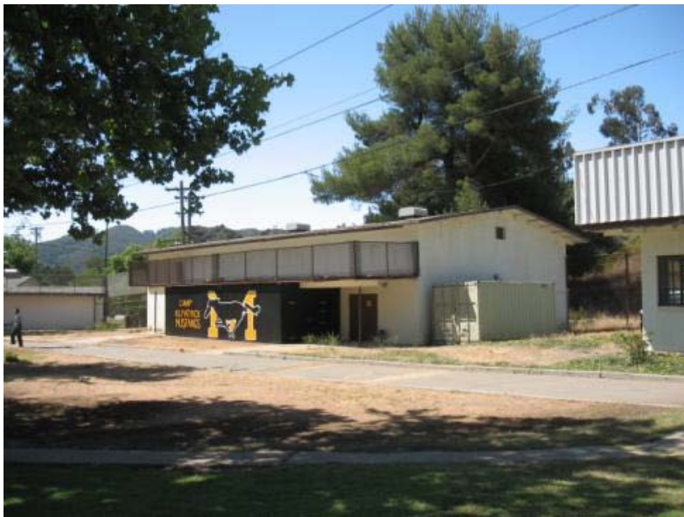
Gymnasium. View looking southwest.
