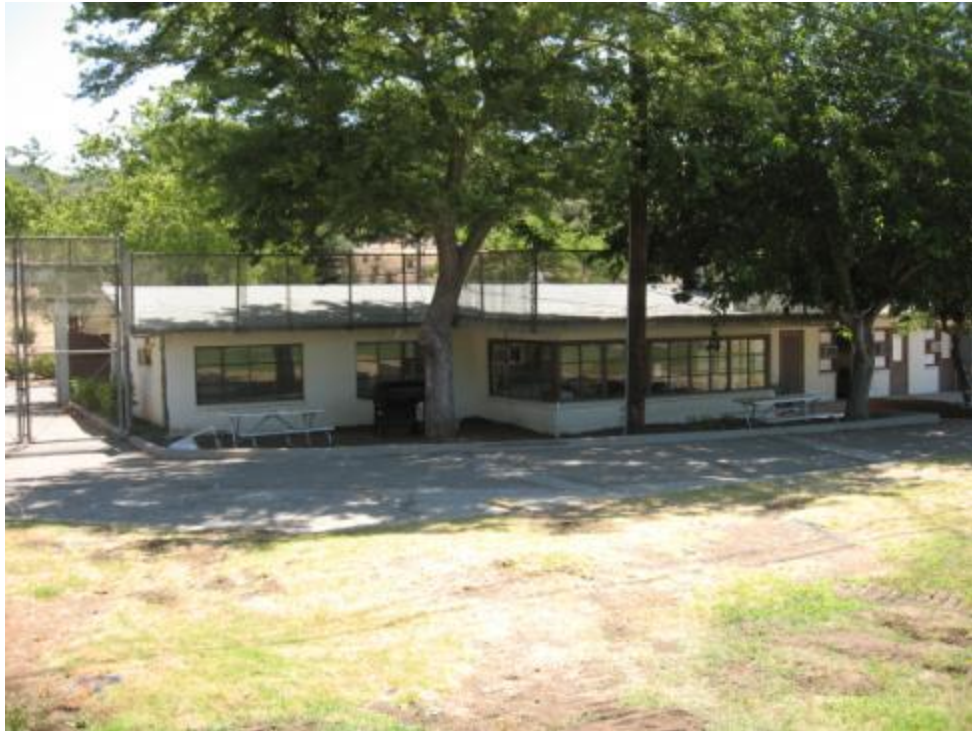
Photograph 10: West elevation of Administration Building. View looking east.
