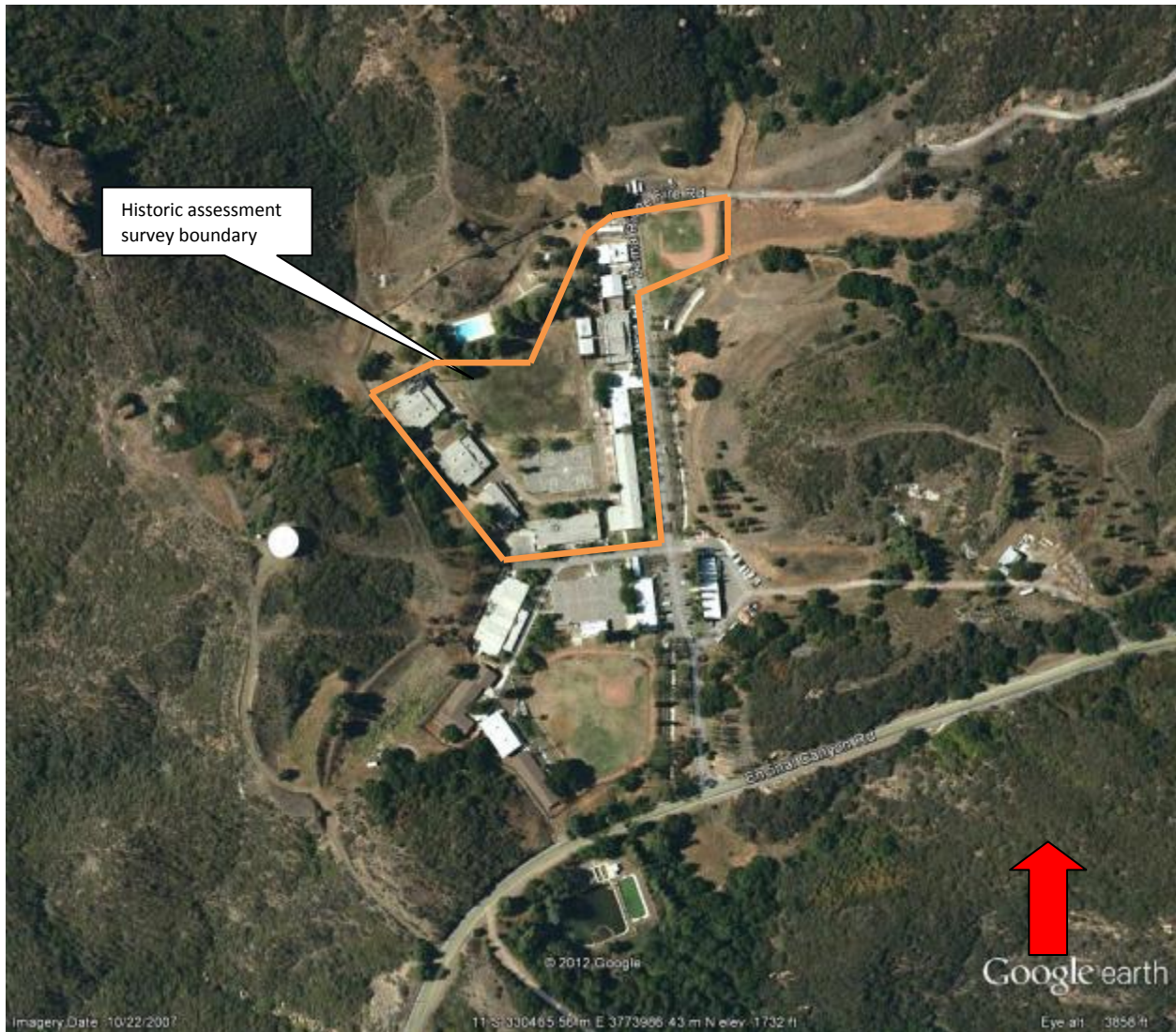
Photograph 1: Aerial view of the buildings and outdoor facilities of Camp Kilpatrick Juvenile Detention Complex being evaluated within the proposed project area.. The Camp Miller complex is located to the south of Camp Kilpatrick, and is outside of the area of potential effect. (Source: Google Earth, 2012)
