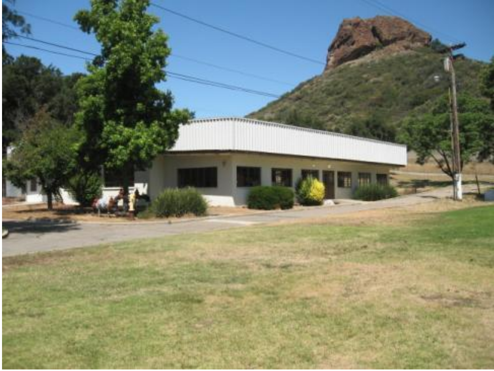
Photograph 5: 40-Bed Dormitory 1A. View looking northwest.
