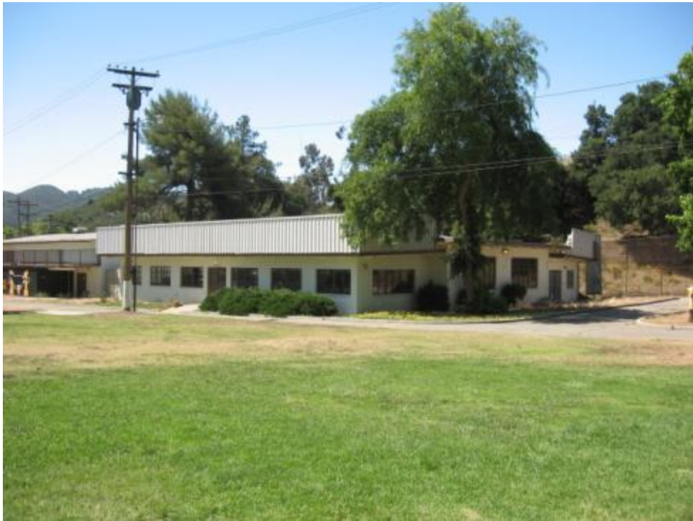
Photograph 6: 40-Bed Dormitory 1B. View looking southwest.
