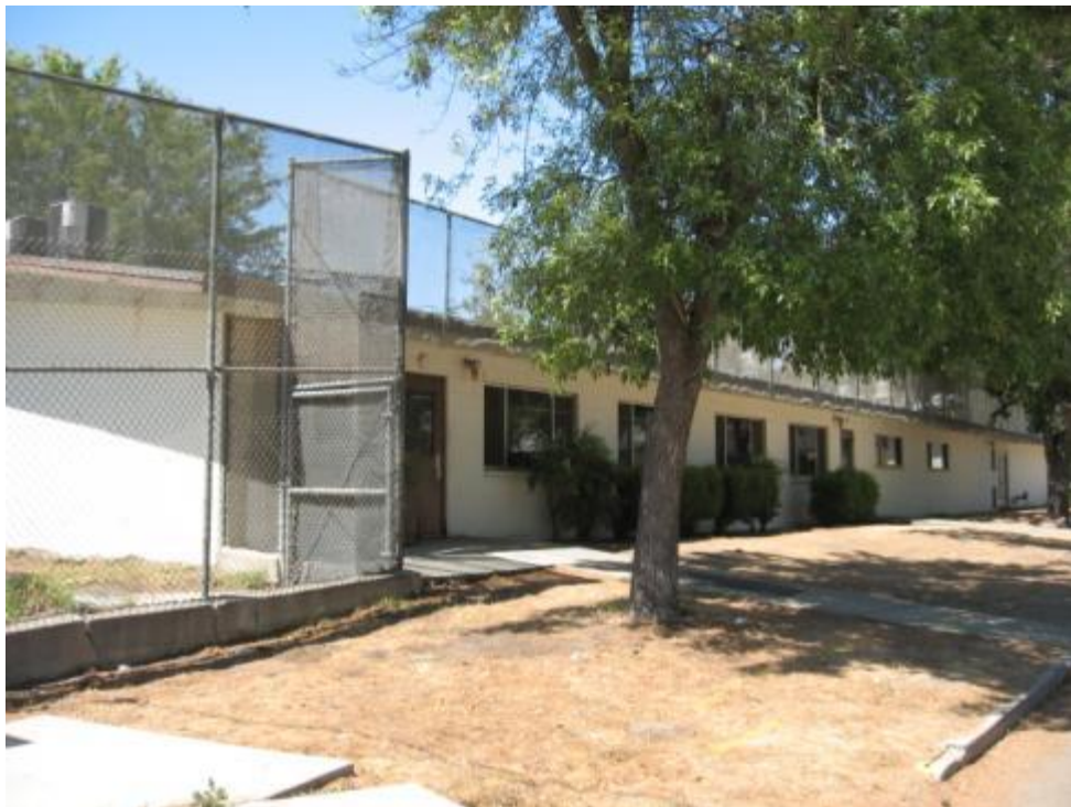
Photograph 8: Shared Kitchen and Mess Hall. View looking west.
