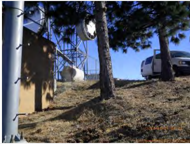
Site view looking north
