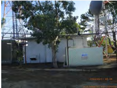
Site view looking north
