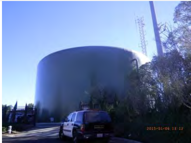
Site view looking north
