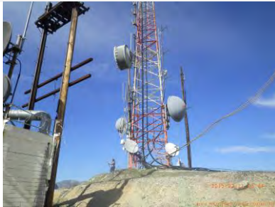
Site view looking north
