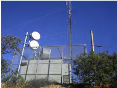
Site view looking north
