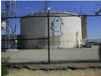
Site view looking north
