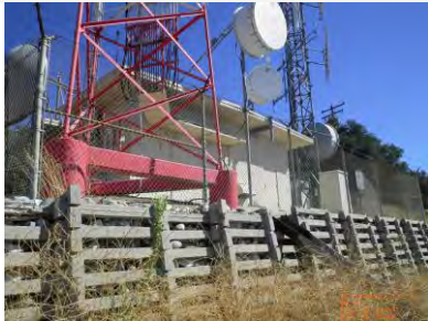
Site view looking north
