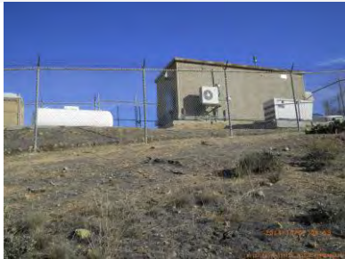
Site view looking north
