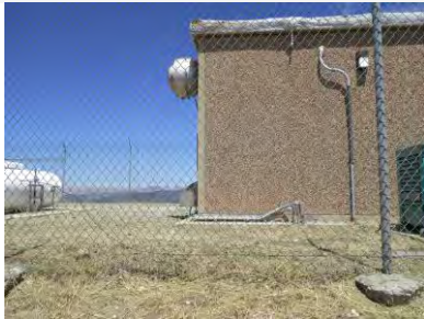
Site view looking north
