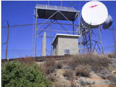
Site view looking north
