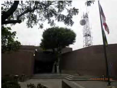
Site view looking north
