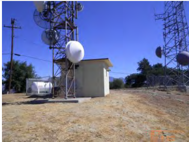
Site view looking north
