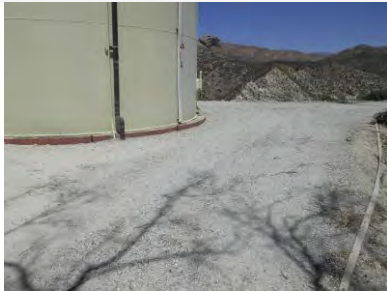
Site view looking north
