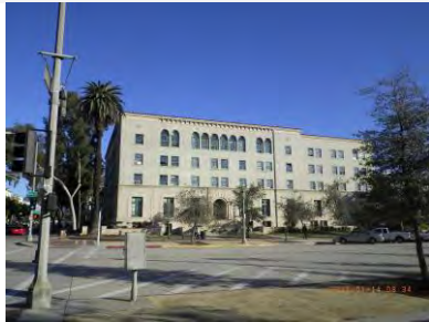
Site view looking north
