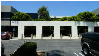
Site view looking north
