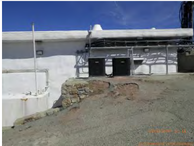
Site view looking north
