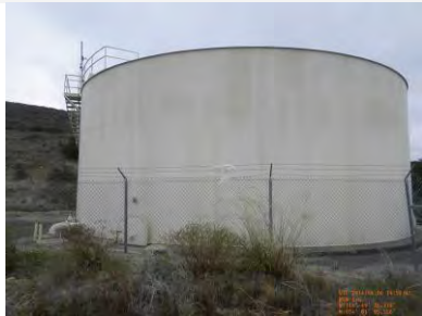
Site view looking north
