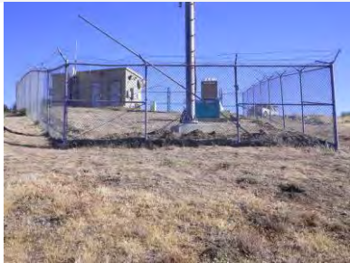
Site view looking north
