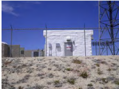
Site view looking north
