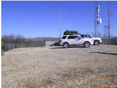
Site view looking north
