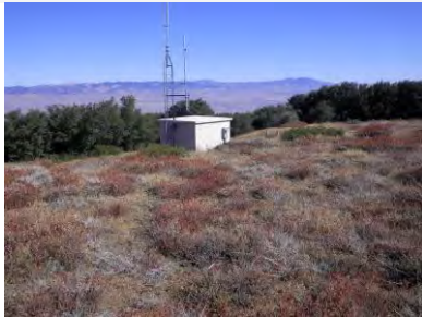
Site view looking north
