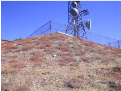
Site view looking north
