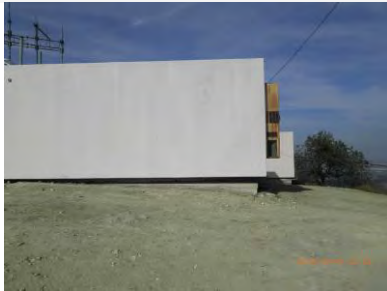
Site view looking north
