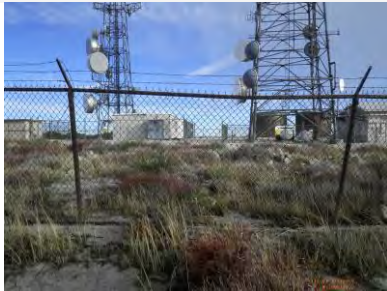
Site view looking north
