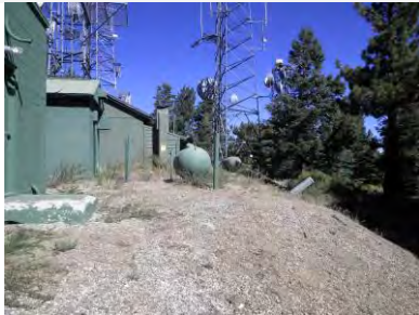
Site view looking north
