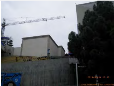
Site view looking north
