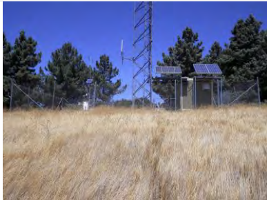
Site view looking north
