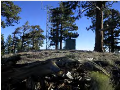
Site view looking north
