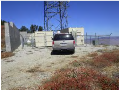
Site view looking north
