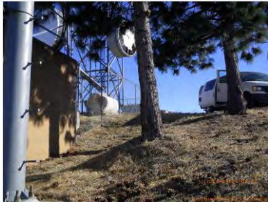
Site view looking north
