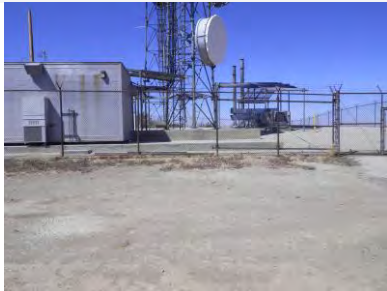
Site view looking north
