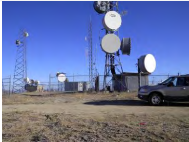
Site view looking north
