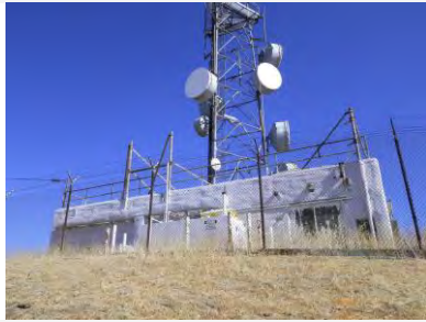
Site view looking north
