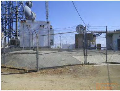
Site view looking north
