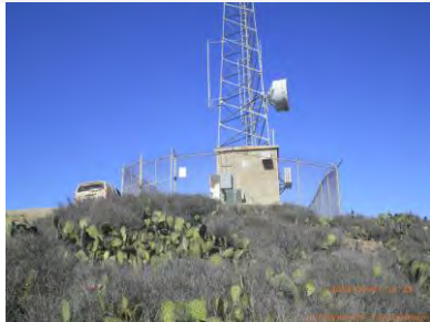
Site view looking north
