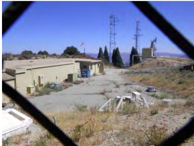
Site view looking north
