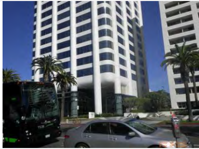
Site view looking north
