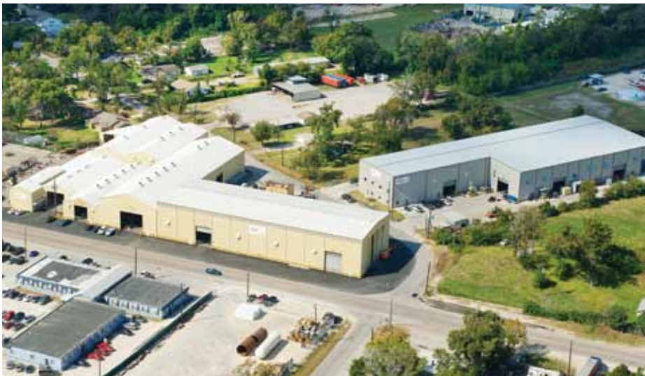
Valve Manufacturing, Houston, Texas
