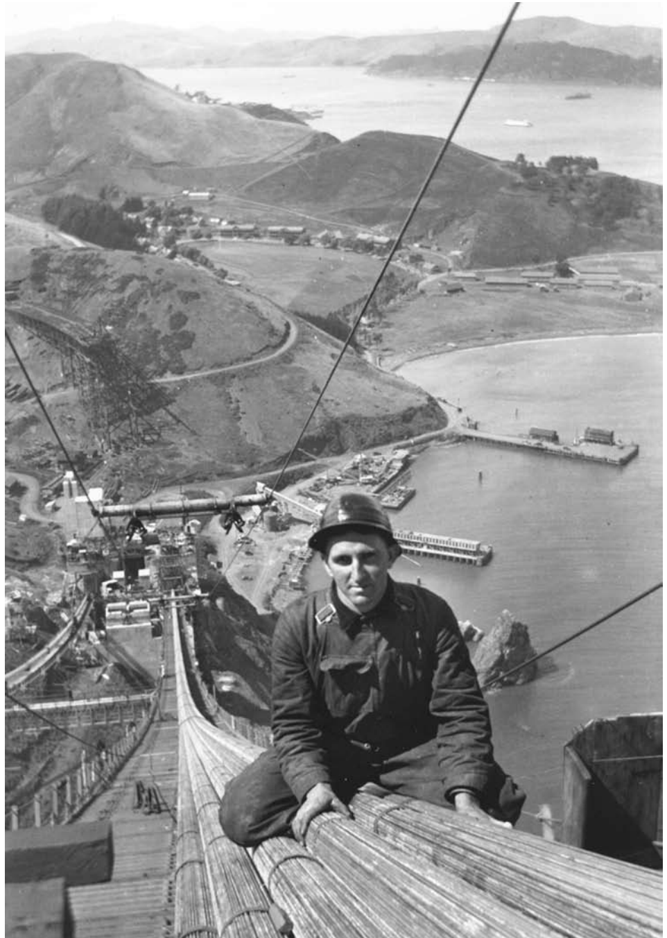
Electrician Fred Brusati, atop the Golden Gate Bridge during construction. (Labor Archives & Research Center)
