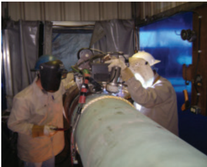
Insituform Technologies will provide corrosion and concrete weight coatings, plus double joint welding, on a new hydrogen pipeline in the Gulf Coast. Shown are the company's pipeline welding services in action. (Photo courtesy of Insituform Technologies, Inc.)
