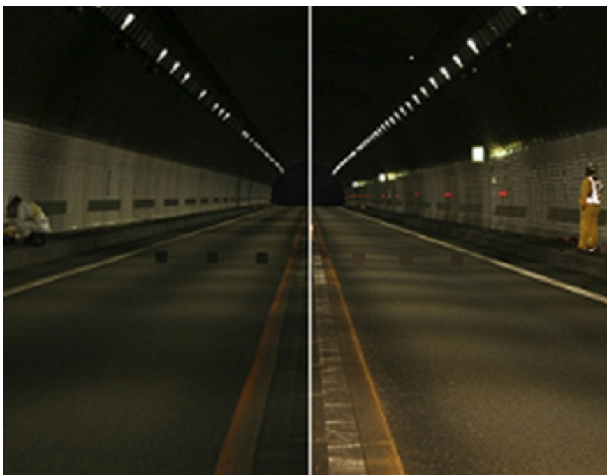
Figure 2 - Tunnel lighting (left: when headlamp is off, right: when headlamp is on, fluorescent lamp)
