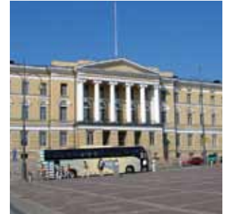
Main university building
