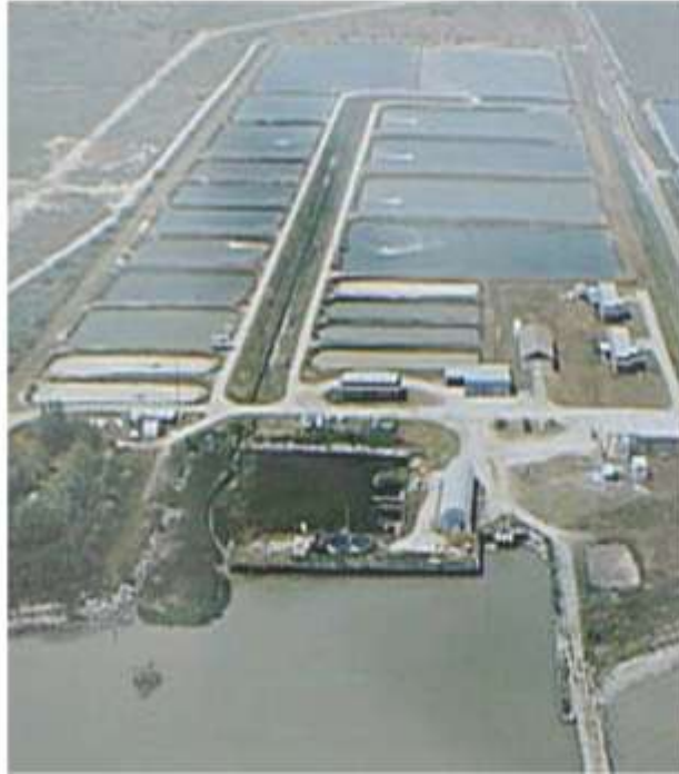
Aerial of Perry R Bass Marine Finfish R&D Facility
