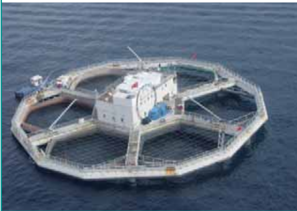
FIGURE 15 A floating fish farm platform fitted with six large cages and a central 2-story work building (Naples, Italy).
