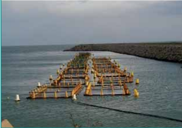
FIGURE 12 HDPE self-built floating cages measuring 7x14 equipped with automatic feeder system (pipes are visible)
