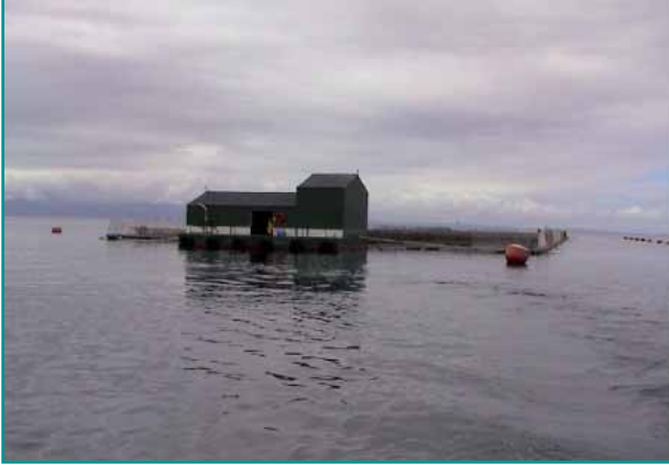
FIGURE 9 Floating barge/house in cages with crew accommodation and feed storage area
