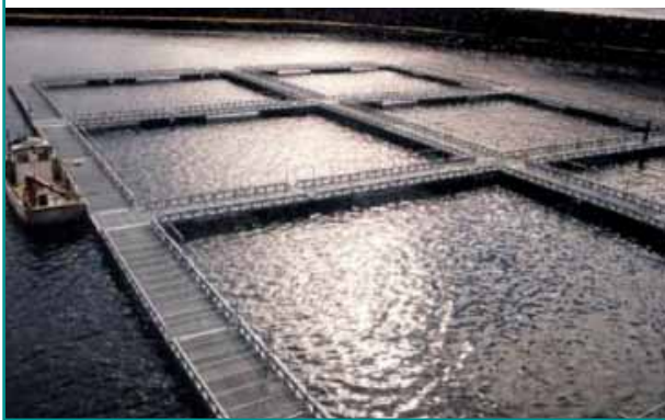
FIGURE 12 Example of steel collar cages
