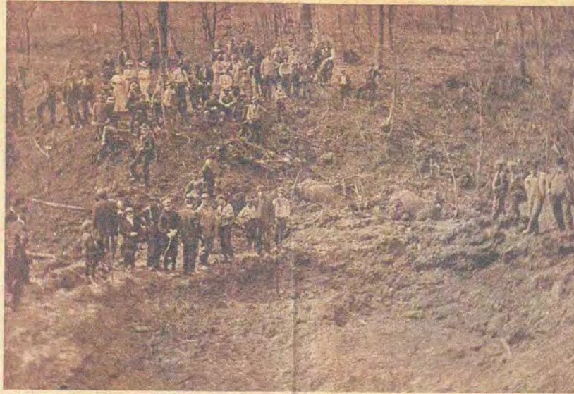
The above picture gives some idea of the havoc wrought by the explosion. The magazine stood in the lower right hand corner, though the picture does not do justice to the huge hole driven in the ground. Near the center of the picture can be seen the bodies of the two horses, their heads being doubled up under them.
