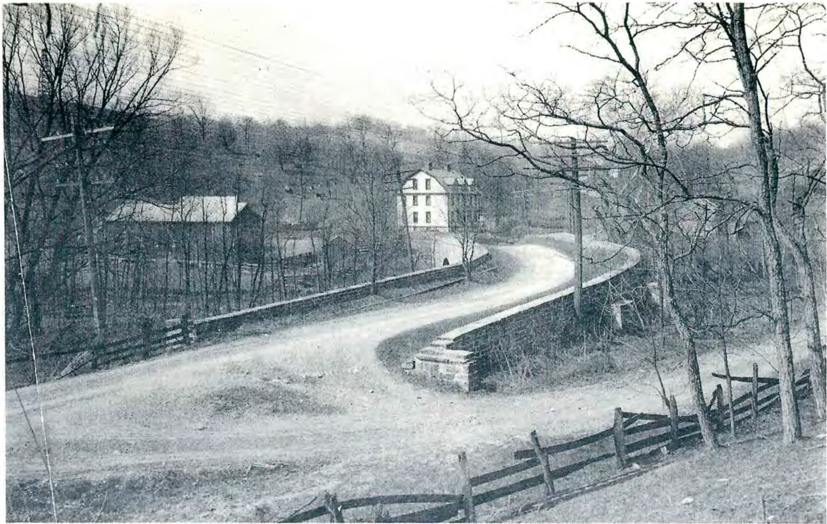
The "S" Bridge, 6 Miles West of Washington, Pennsylvania
