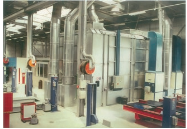
Building of a truck service center in Iraq
