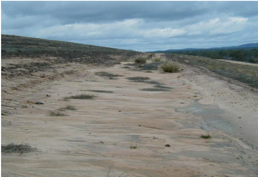
Figure 1. A 5m wide berm that has become filled with sediment one season after construction.
