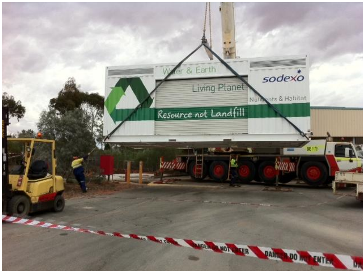
Figure 3: GaiaRecycle G-1200H being delivered in customised Sodexo modular housing to Olympic Dam Village rear kitchen dock.
