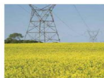
Upgraded electricity grid
