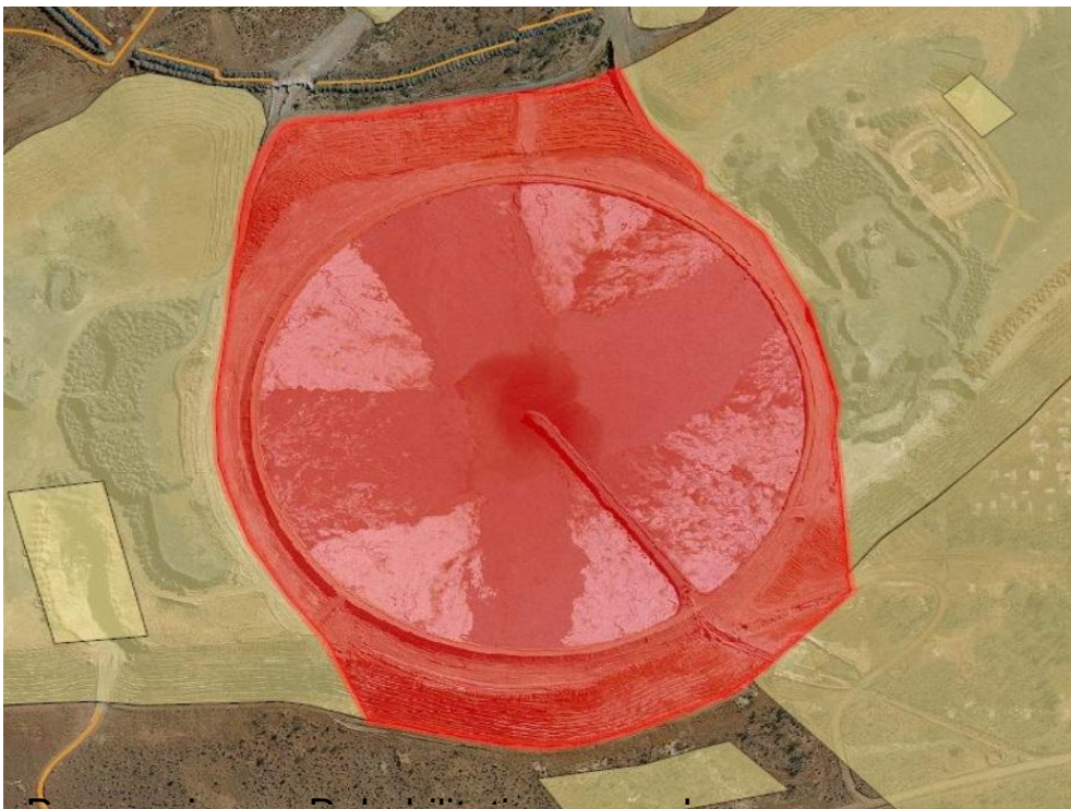
Figure 2: Tailings Storage Facility highlighted within the PRAC™ (Progressive Rehabilitation and Closure) System at Challenger mine site.
