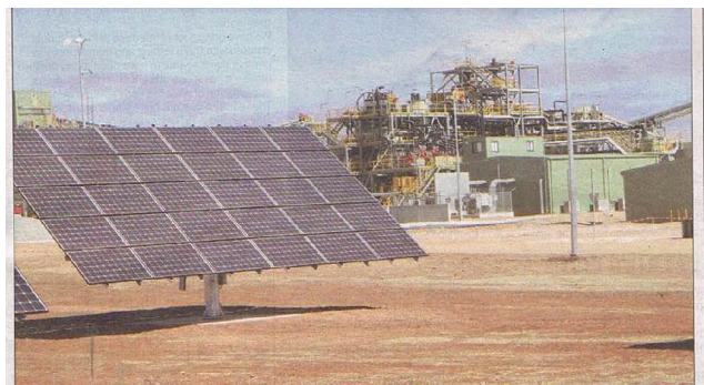
GALAXY Resources' Mt Cattlin mine is in the process of becoming Australia's first, renewable energy-powered mine.
