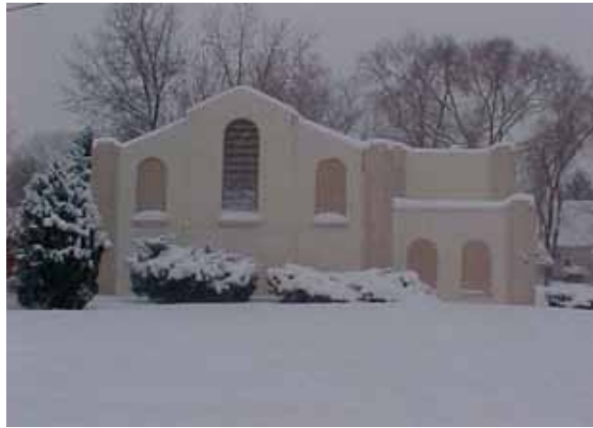
FIGURE 2-2 Sandstone Well No. 3 in Waukesha
