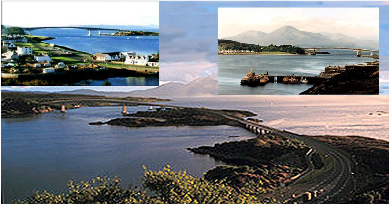
The Skye Bridge from E
