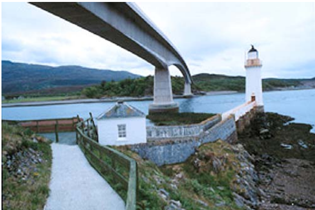
Kyle Akin Light (disused) and the Skye Bridge from W
