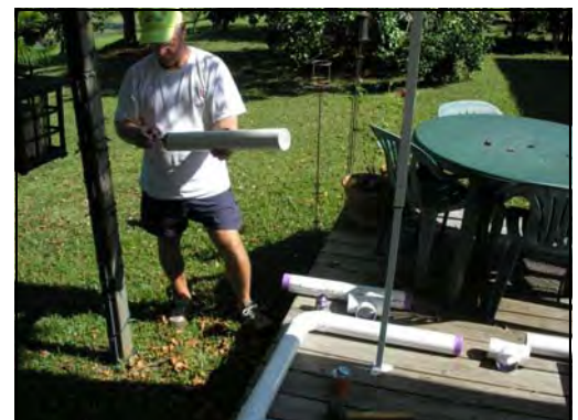
Jim Smith cleans the pipe in preparation for assembly
