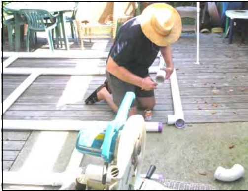
Don Hardy gluing pipe components together
