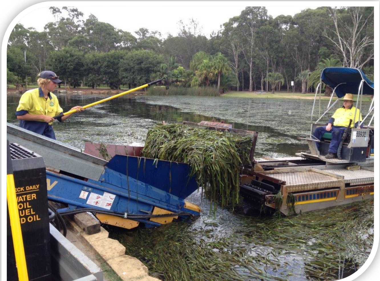
Aquatic Weed being managed in Woodcroft Lake, Blacktown
