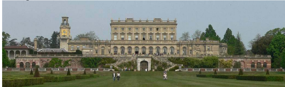
Cliveden House, with the balustrade in the foreground
