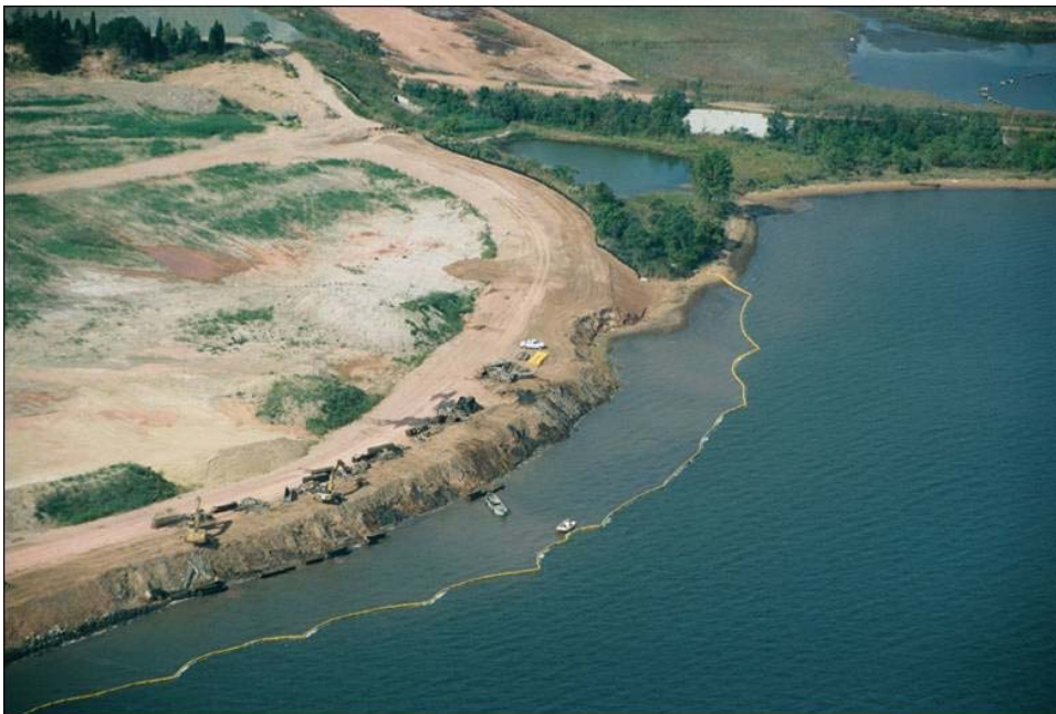
Figure 51: Example of a Turbidity Control Barrier for In-Water Placement Of Dredged Material
