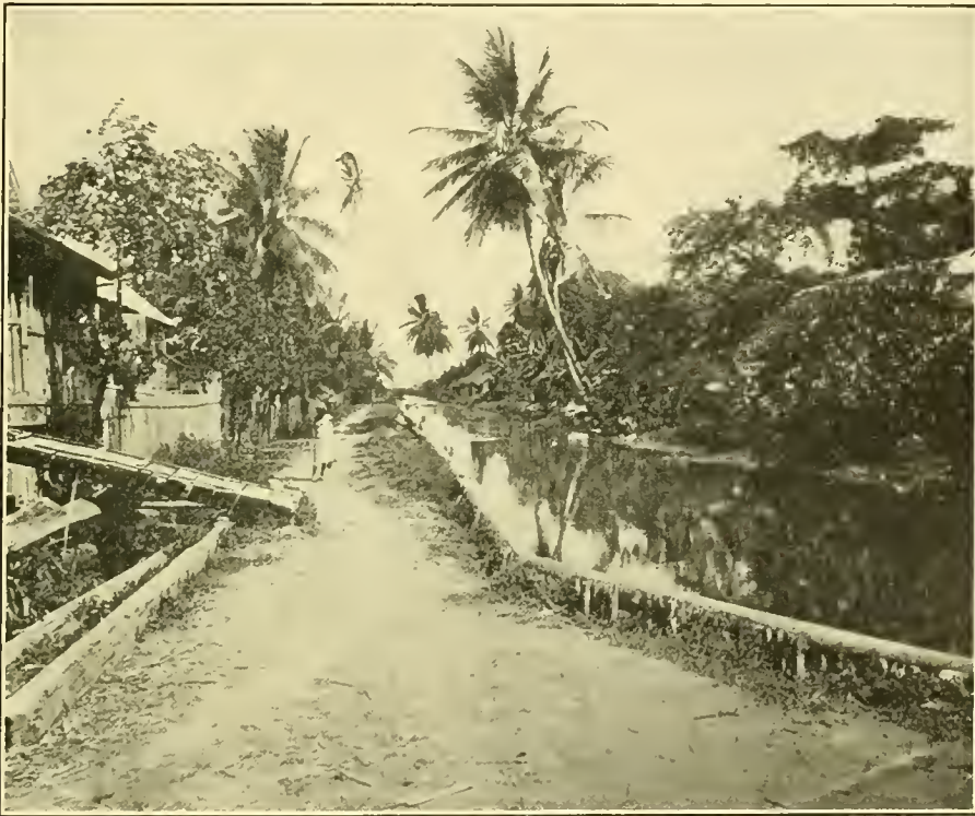
FIG. 4. View of the drainage canal at Cane-Grove Corner.
