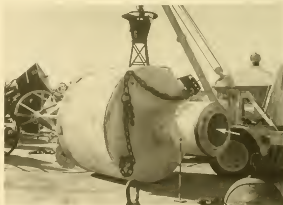
FIG. 1. Typical navigation buoy. Arrow indicates the sheltered, inner portion of the stabilizer tube.
