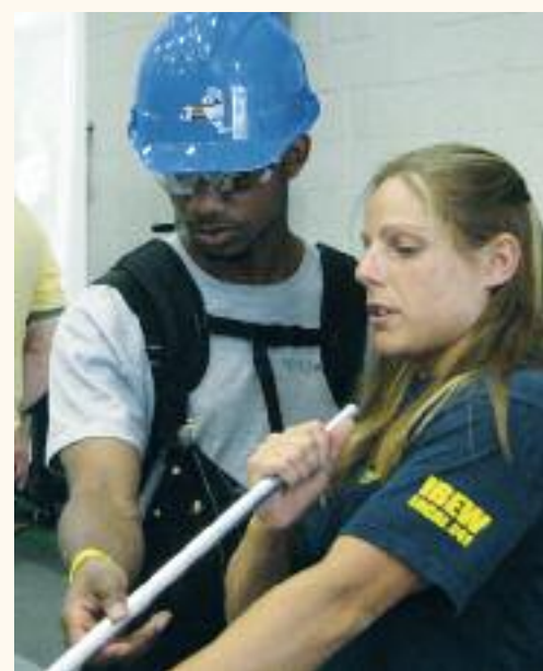
Ithaca, N.Y., Local 241 journeyman Kathryn Boucakis instructs a student in pipe-bending at a Central New York Careers in Construction Day event.
