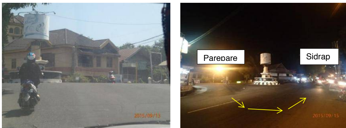
Figure 4-8 Road intersection. The turning corner is hairpin curve and uphill road
