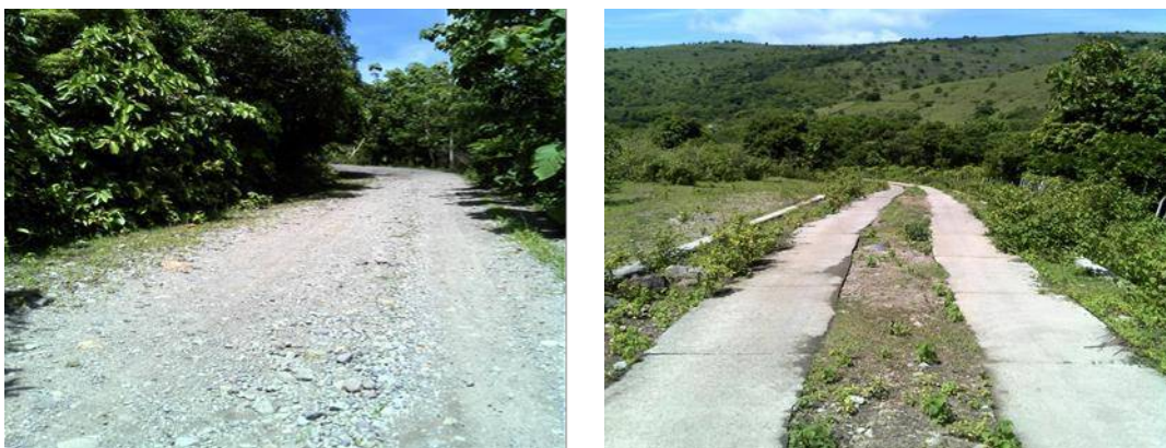
Figure 4-12 Access Road Connecting Mattirotasi Village to Site
