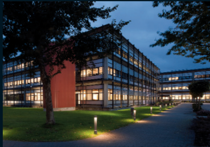
Statoil headquarters, Stavanger. Lighting design: Statoil ASA.
