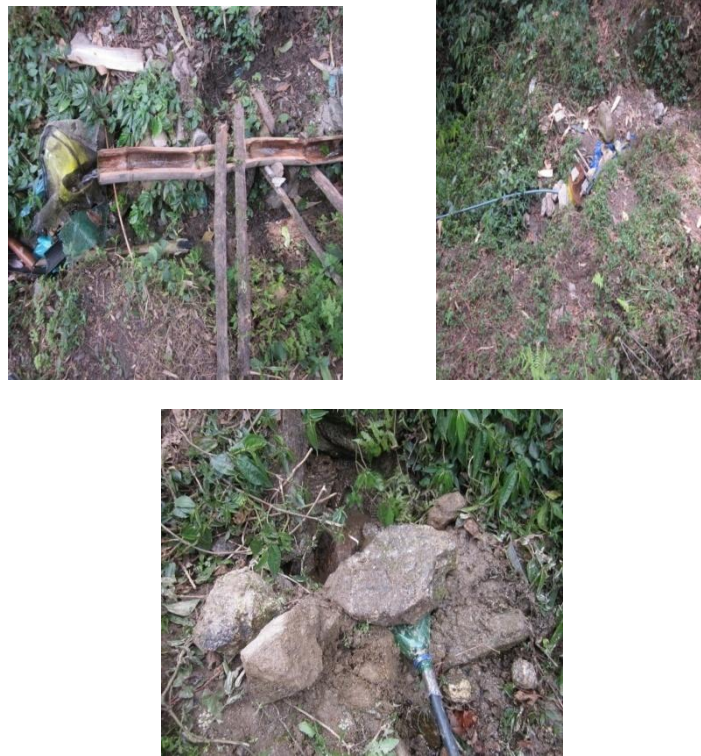
Figures: 33 (a, b, c) : Local technique to carry water from Source so called “kua or muhan” by which water is being collected to a big container called Thumbhi (Large reservoir) and from there supplied to Village via a pipeline for a kilometer or more to carry water by the help of pillars of Trees in the hill slopes. First figure indicates Thumbhi, second and third figure for kua. Note that bamboos (half pipe) are used to carry water from Hills.
