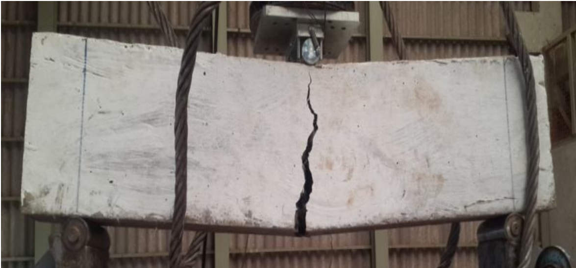
Plate 4.9: Failure pattern of L.B.740 beam
