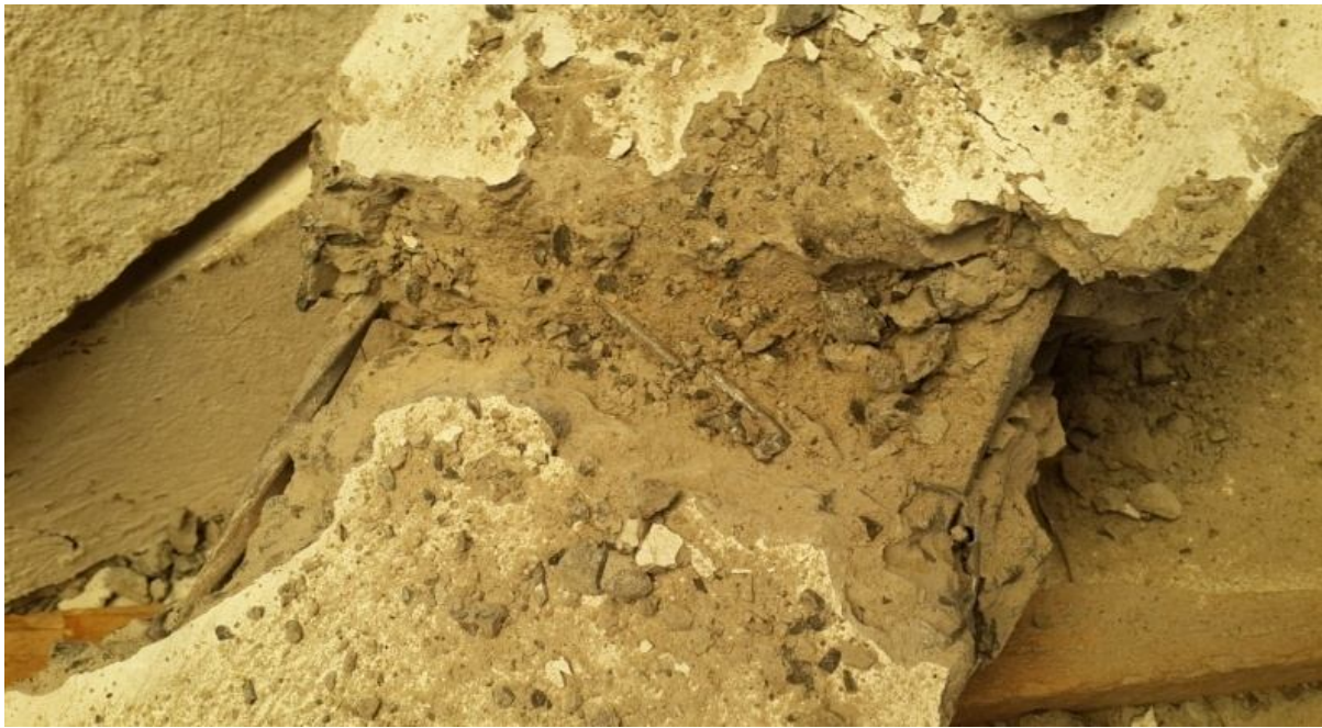
Plate 4.21: unbroken shear reinforcement for Steel 1x6 beam
