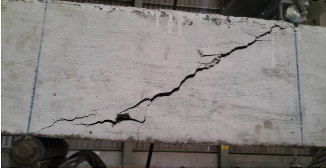
Plate 4.14: Failure pattern of L.B.1x6 beam
