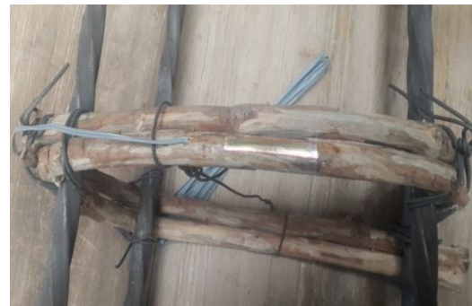
Plate 3.9: Fixed shear reinforcements
