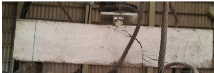
Plate 4.18: Failure pattern of L.B.2x10 beam
