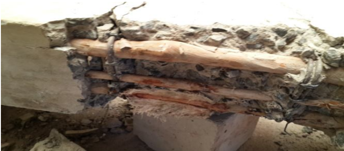
Plate 4.25: unsnapped L. buchananii tensile reinforcement
