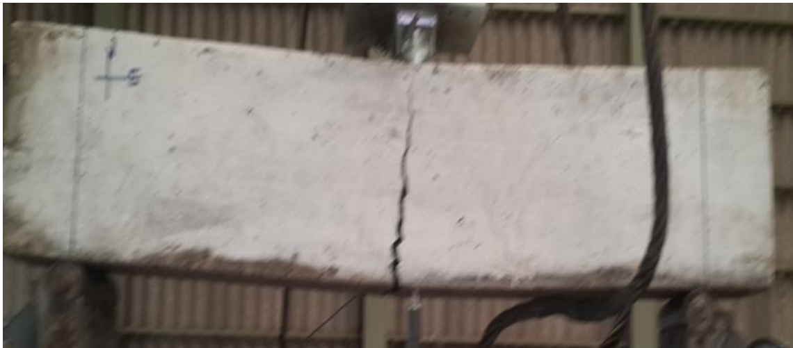
Plate 4.7: Failure pattern of L.B.787 beam
