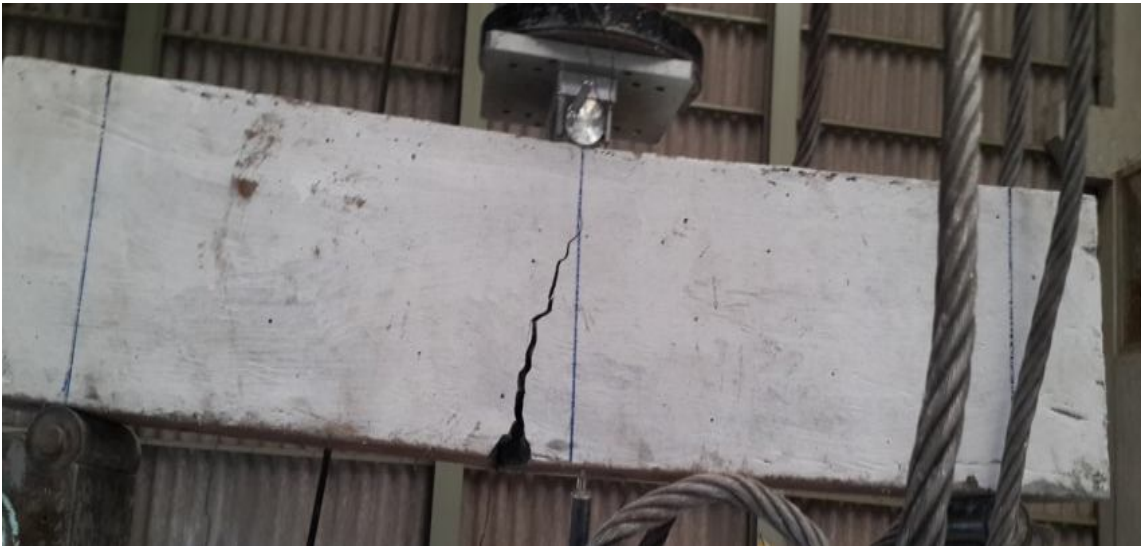
Plate 4.22: Failure pattern of Steel 1x6 beam
