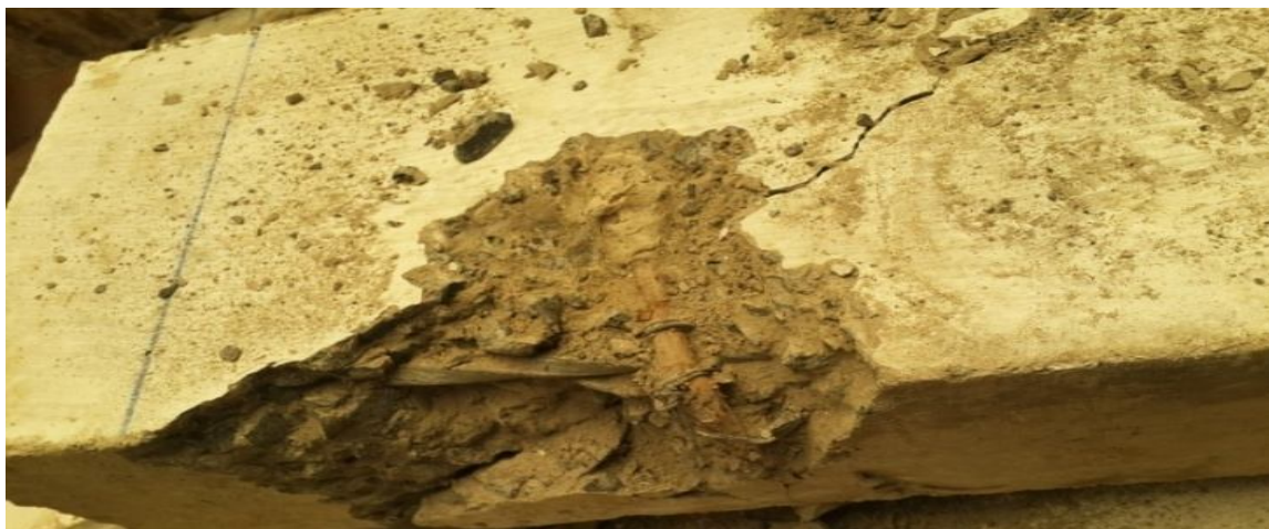
Plate 4.15: unbroken shear reinforcement for L.B.1x8 beam
