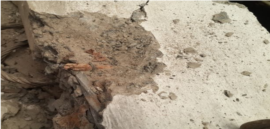
Plate 4.13: unbroken shear reinforcement for L.B.1x6 beam
