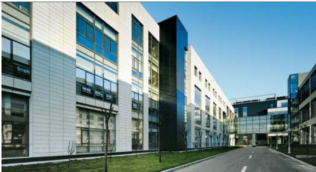
Centrin Data Centre, Beijing/China
