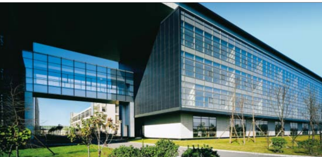
Centrin Data Centre, Beijing/China
