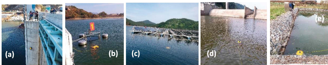
Fig. 2. Underwater structure by ROV and (a) Dam, (b) water circulation system, (c) floating solar power plant, (d) multi-function weir, and (e) sediment sites.
