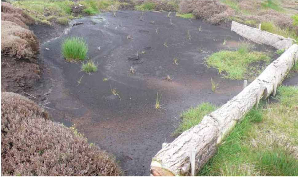
Figure 7. Dams constructed with Lawson Cypress trunks in small streams to promote peat retention and its revegetation.
