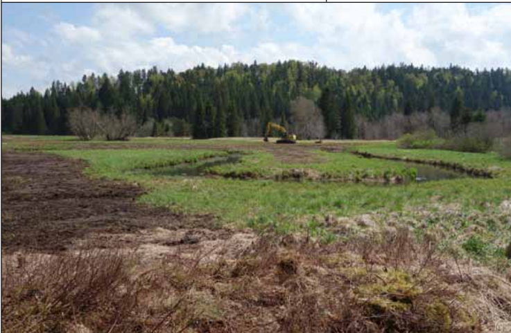
Figure 9. Restoration of drainage before refilling.
