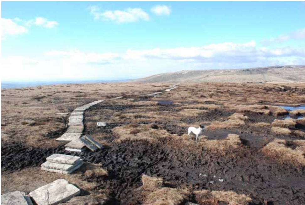
Figure 7. Flagstone footpath installation across moorland eroding due to visitor traffic.
