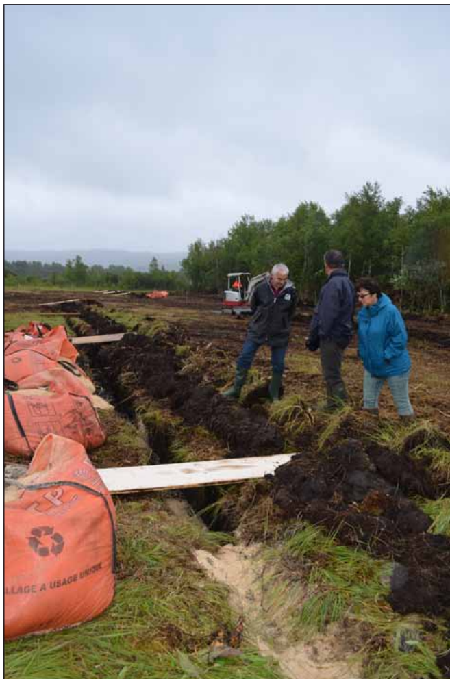
Figure 6. Restoration of drainage before refilling.
