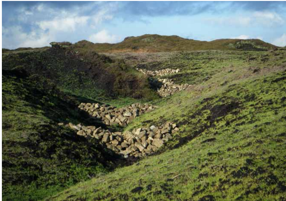
Figure 5. Semi-permeable stone dams limit sediment transport and slow stormflow from the moors.
