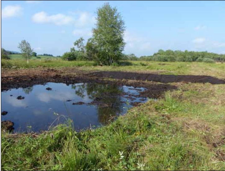
Figure 4. Blocking dam and peat covering.
