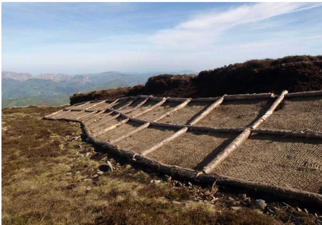
Figure 6. Protection of the bog slopes with coconut fibre matting.
