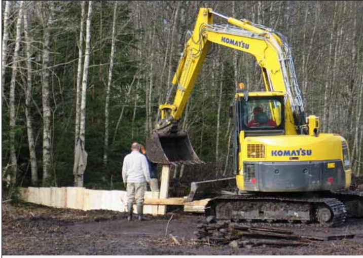
Figure 12. Construction of a dam.
