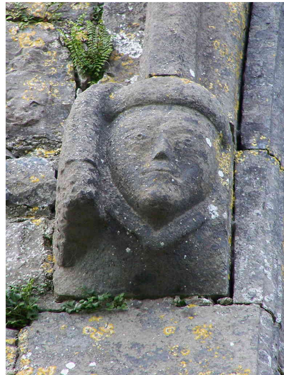
Figure 6 Carved head label-stop on the southern side of the east window of Rosserk friary
