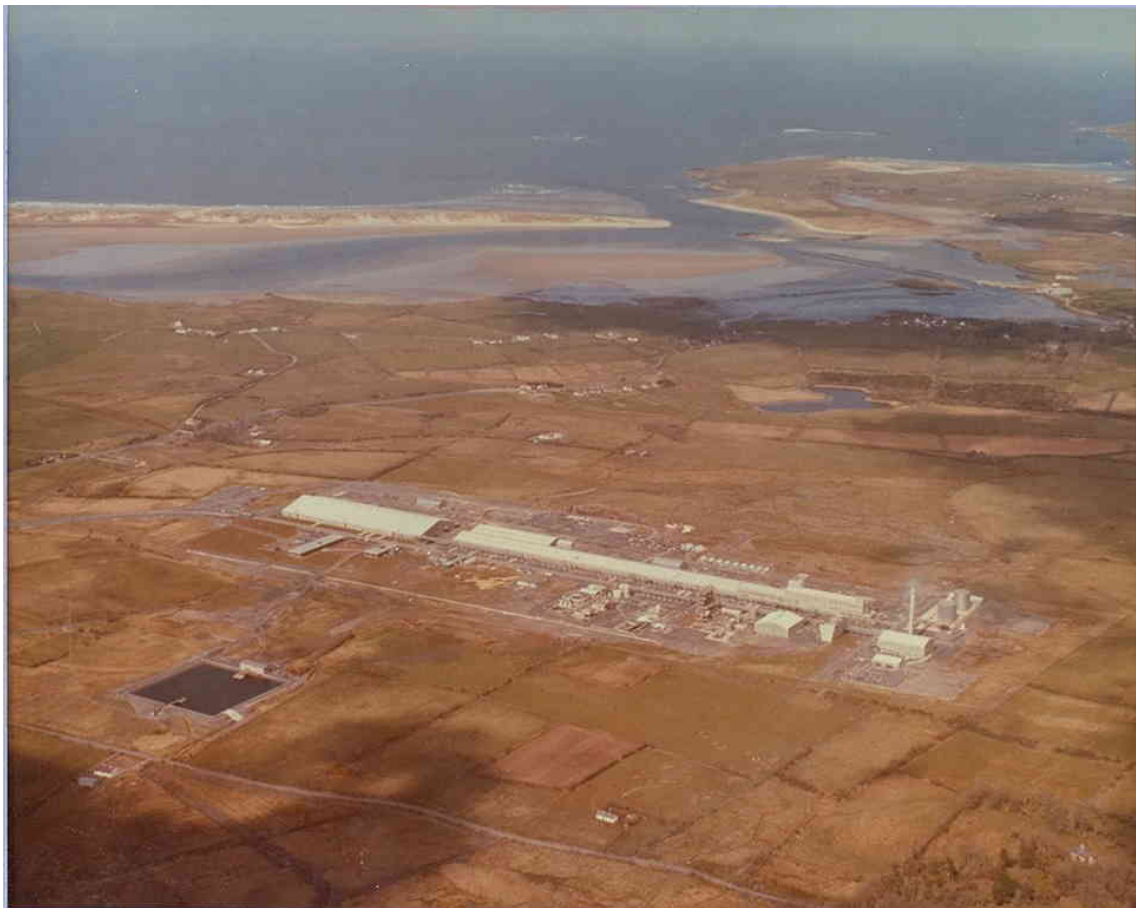
Figure 1 Asahi factory on completion in 1977
