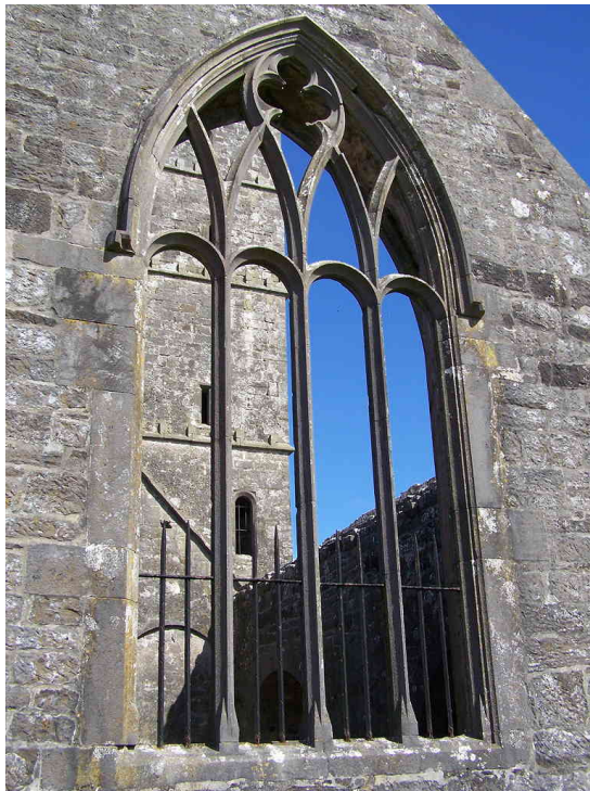
Figure 5 Switchline tracery window in the south wall of the transept of Moyne friary
