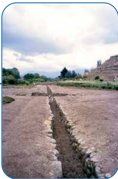
Cuenca: remains at Pumapungo of an ancient water system from the Inca city of Tumipamba, Ecuador © UNESCO/Alison Clayson
