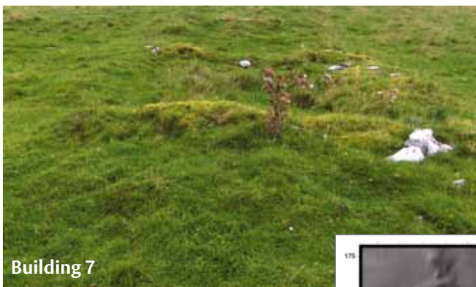
23 Building 7 from the southeast. The scale is on the far gable end
