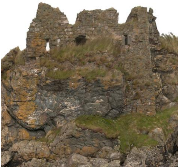
Figure 3 South-facing façade of the hall building at Dunyvaig
