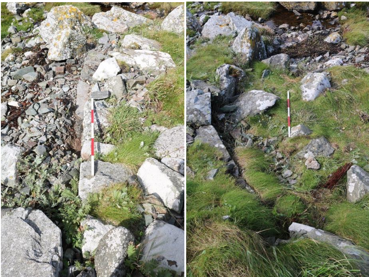
Figure 8 View of the straight outer line (left) and curved inner line (right) of the western bastion wall looking north from the courtyard wall.
